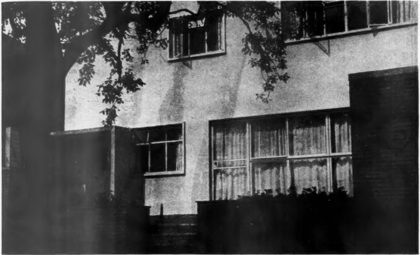
Above, a view of the south-east front.
