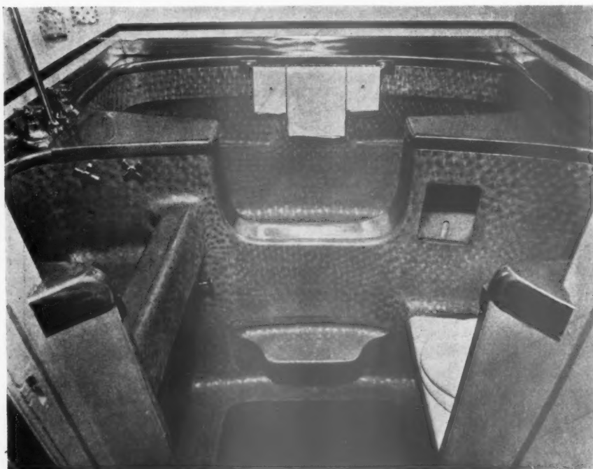
A New York remodelling in which the use of Buckminster Fuller's prefabricated bath unit has allowed two bathrooms in the space formerly occupied by one. [From the "Architectural Forum."]
