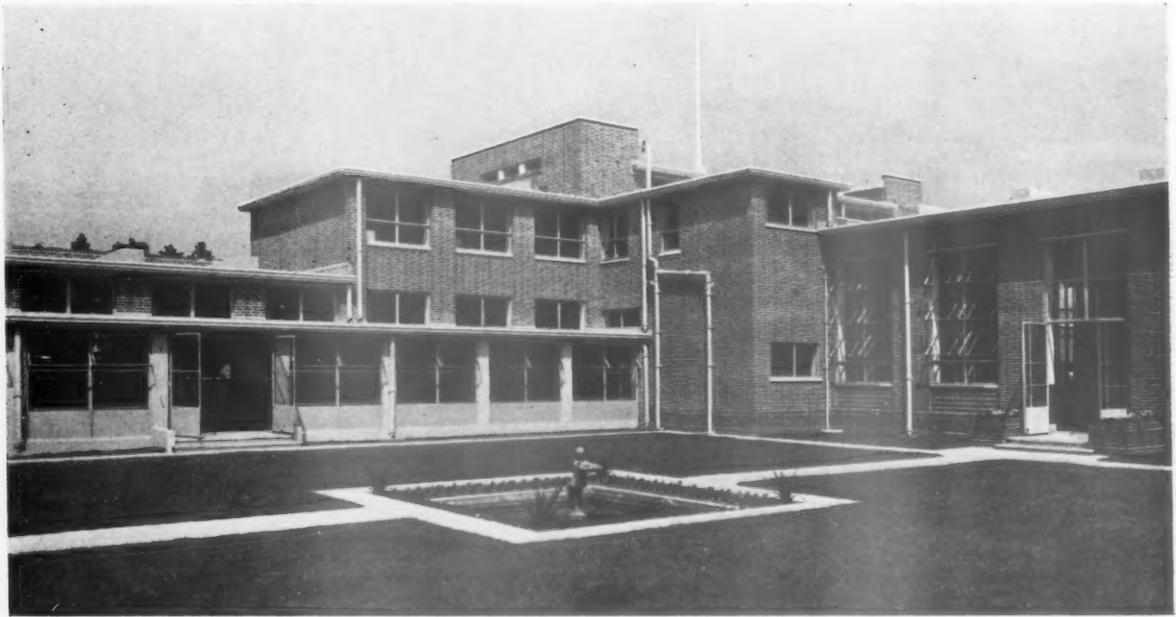
GENERAL AND SITE (cont.)—The main school block has therefore been designed on the quadrangle principle to conserve space, the site has been levelled out for each block of buildings and mass concrete piers with reinforced concrete beams and suspended floors are provided to that part of each building on made-up ground. The
