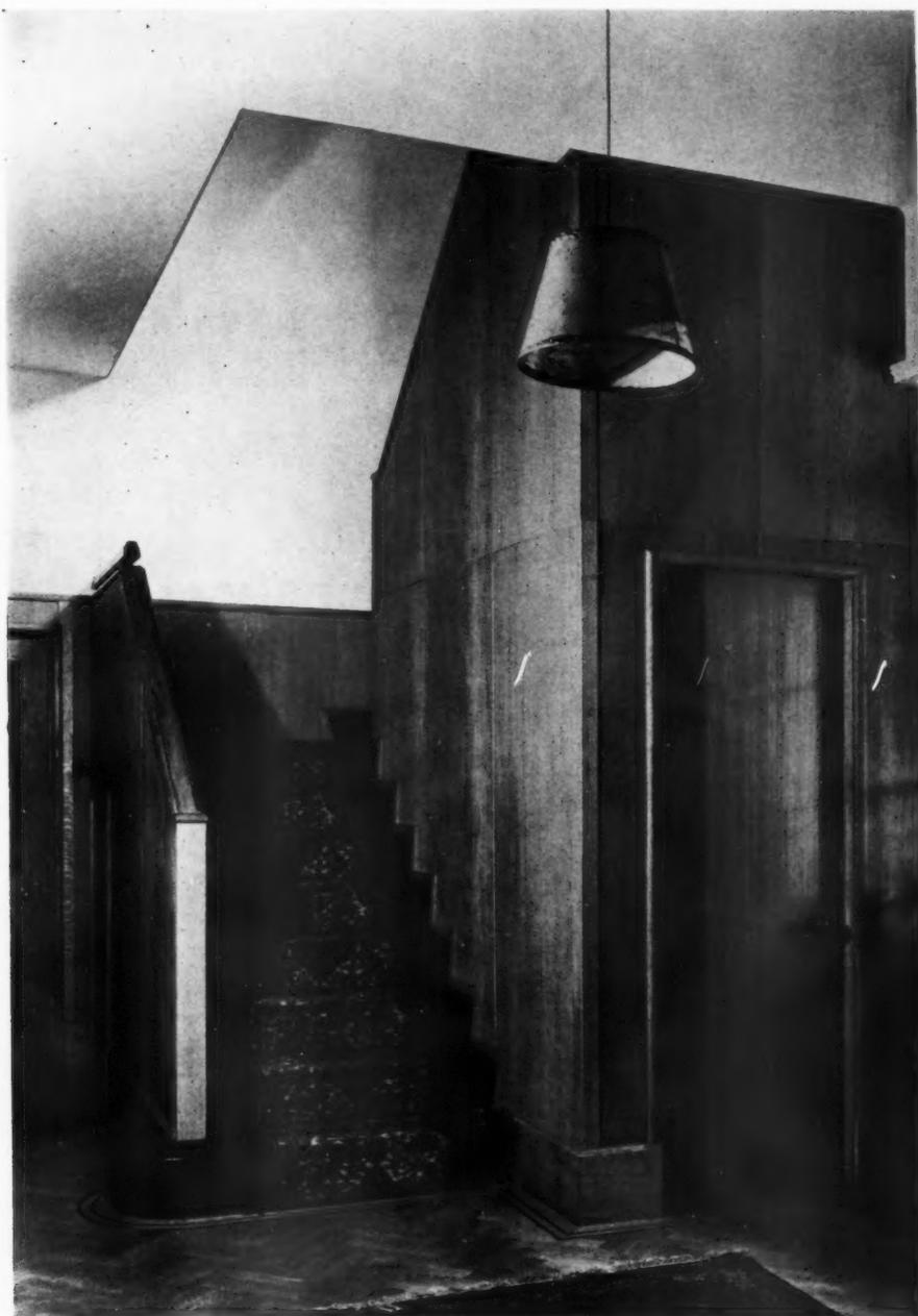
The staircase illustrated has been re-constructed in an existing building. The staircase is constructed in oak, treads and risers being stained black and polished. The balustrading is panelled in oak plywood with V joints, natural finish and wax polished, with cappings and strings in solid oak. Details are shown overleaf.
