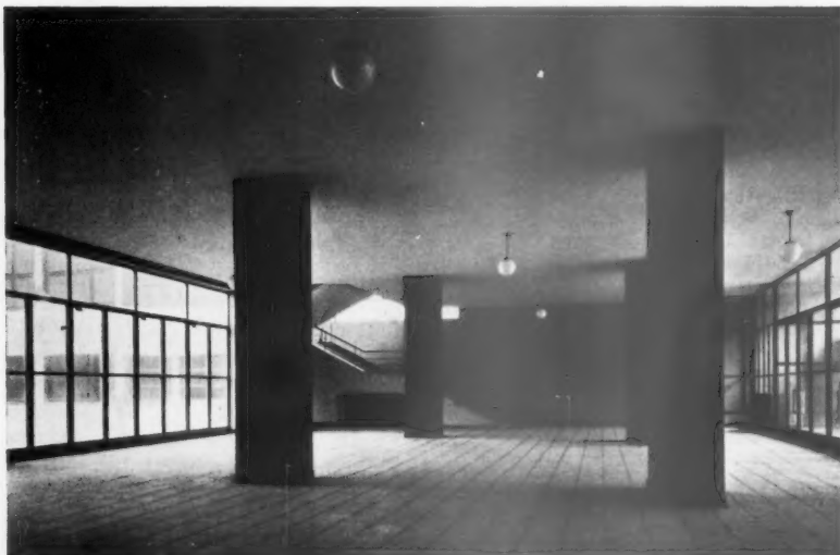
4 : School at Prague, interesting for its open planning and spacious entrance hall with all-opening glass walls, used for play in wet weather. Notice dispersed lavatory planning in main part of school. Architect: Jan Gillar.
