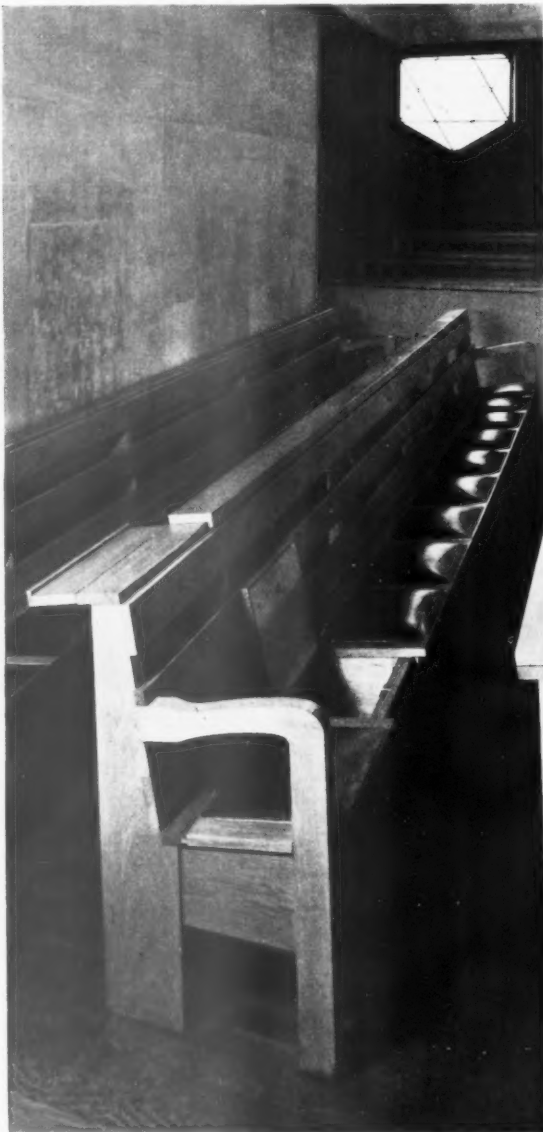
The photographs show: below, a row of seats: beneath each seat is a locker for books; right, one of the Rabbi's seats; and a view of the ceiling beneath the gallery. Above, typical part longitudinal section showing reinforcement to roof slab and tie beam.
