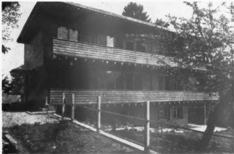
A timber house in Reigoldswil, by R. Preiswerk. [From "Werk's" timber number.]
