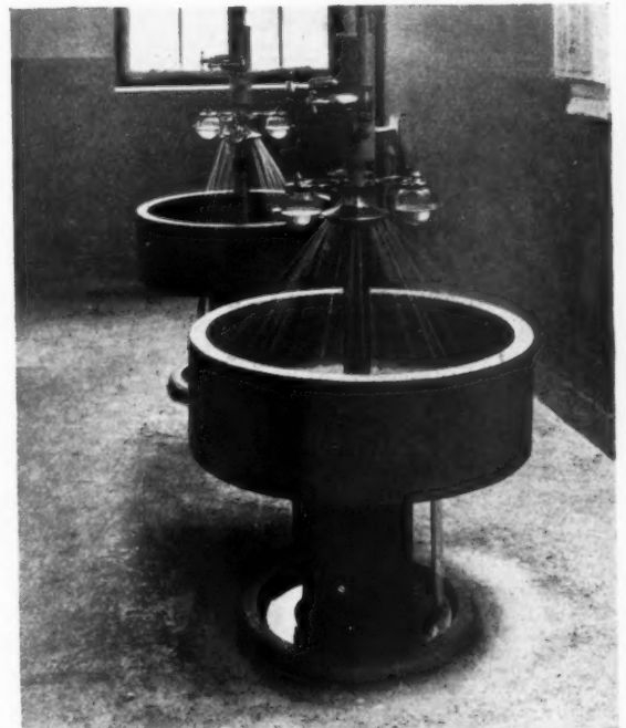
Dimensions and photograph of washing fountains which are being increasingly used in Senior Schools. Water may be either hand or foot controlled.
