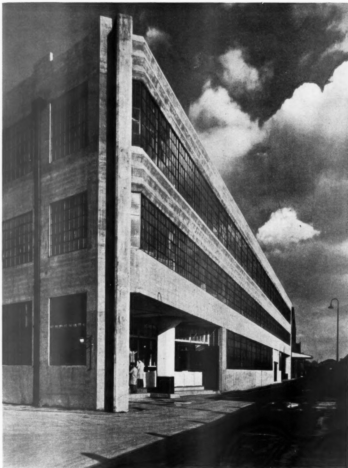
Another view of the machine store. The building is the height. The roof can be used as the floor of an elevated reservoir, with 4 ft. depth of water.
