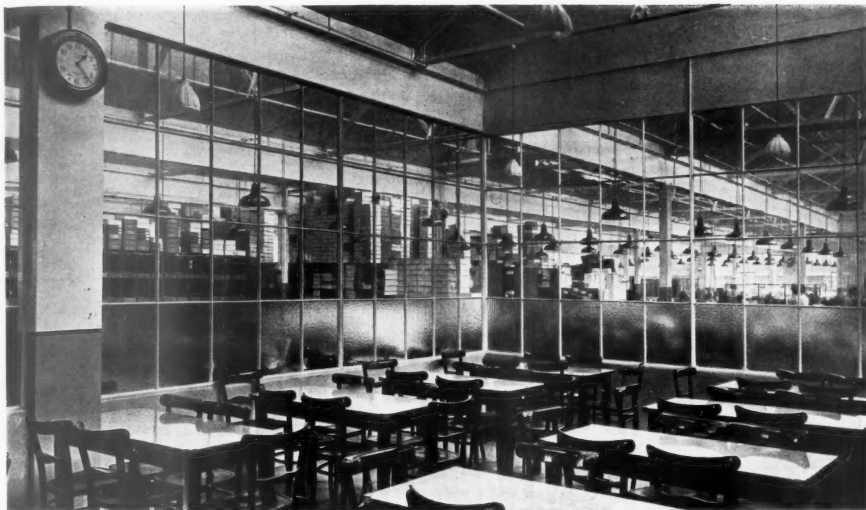
A general view of the canteen in the Jantzen knitting mills, showing canteen furniture and steel partitioning, with industrial lighting reflectors in the works beyond.
