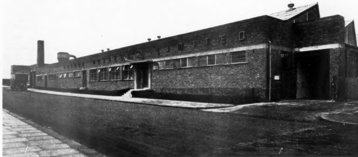
Factory for Gordon Russell, Ltd., Park Royal, Middlesex, for the production of radio cabinets. Architect for the exterior: G. A. Jellicoe. Assistant: M. J. H. Bunney. Layout was to be flexible for easy adaptation to other forms of "clean" manufacture. Construction and finishes: Standard steel factory-type roofing with solid brick walls and all internal partitions movable. The south wall of the low office string was raised both to mask the factory roofing and also to provide a background for the clients' standard sign, and the external treatment had to comply with the standards already arrived at by the contractors on previous work. Brown-red stock brick; concrete steps, string and cills; door surrounds, cement rendered; windows, standard steel casements, painted cream; lettering and sign of wood, save for the circular saw of the sign, which is of steel; faces of the lettering painted cream and the edges bright blue; sign finished in blue, cream and grey.
