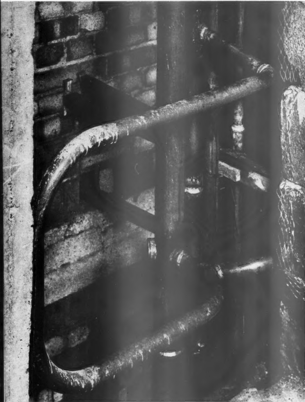
This close-up view of the installation was taken after the erection of the dividing wall between the kitchens, and shows the various bronze welded joints in the main stacks and branches. The welded cleaning eye on the waste stack can be seen behind the point of entry of the combined wastes from the sinks, while one of the holderbats beneath a weldable socket fitting is visible on the main vent shaft. The bronze welded water service pipes are on the right-hand side.
