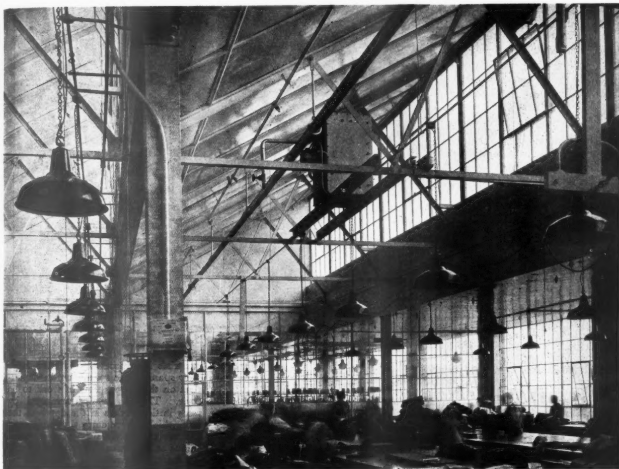
Roof steelwork and vertical northlights at the Jantzen knitting mills.
