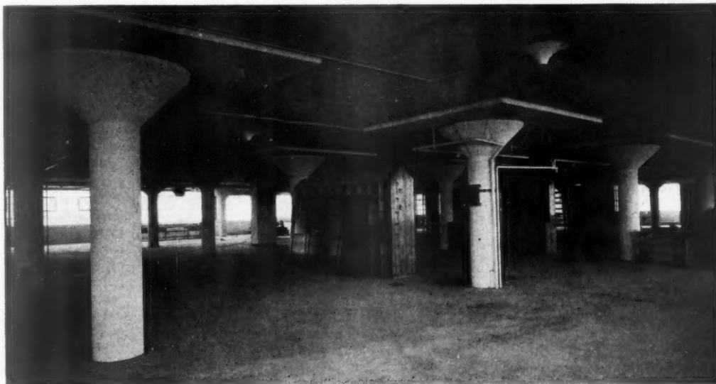
Mushroom columns in a reinforced concrete multi-floor building. J. L. Cowes and Partners, architects. Note radiant heaters slung from the ceiling.
