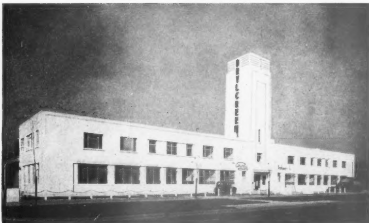
Factory on the North Circular Road, N.W.10, for County Perfumery Limited. Architects: Nicholas and Dixon-Spain. A steel-framed building with brick infillings.
