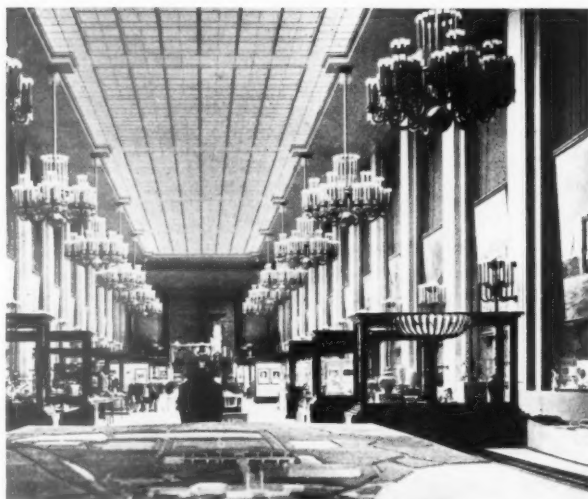
The interior of the German pavilion at the Paris Exhibition. The illustration is interesting as showing the latest developments in German architecture. The photograph is by courtesy of the Exhibition authorities.
