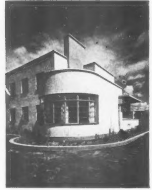
The photographs show: left, the cubicle block; above, the bay window to the matron's sitting-room; below, one of the pavilions for particular diseases.
