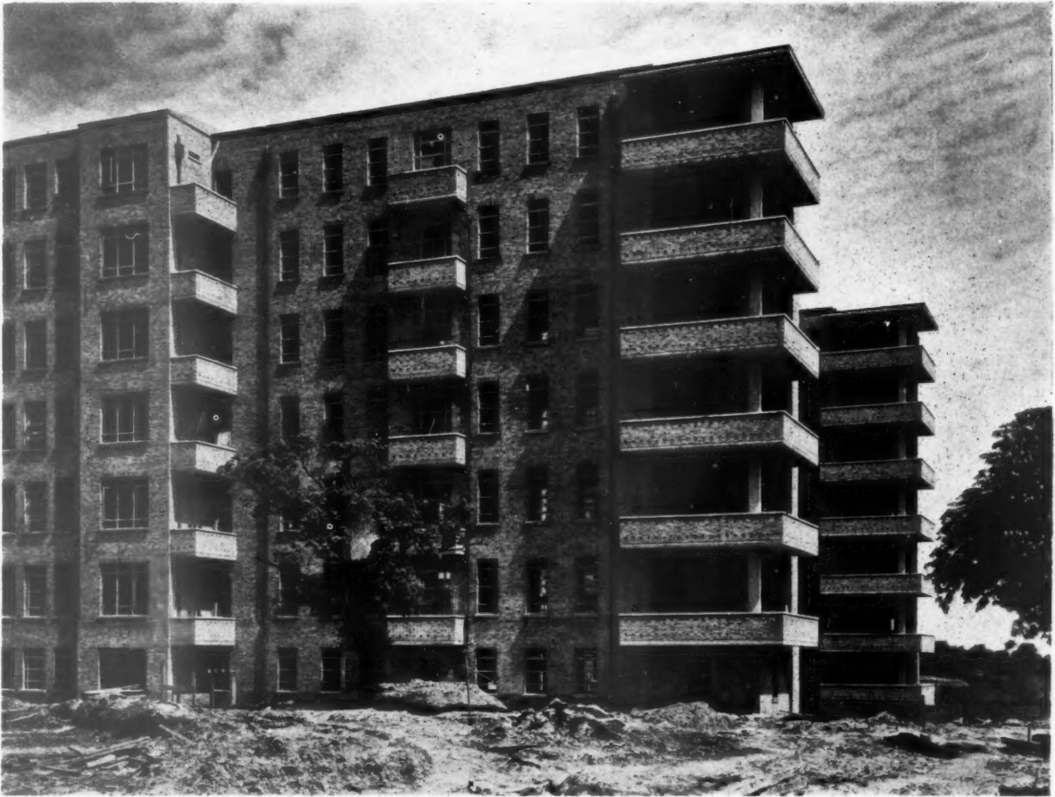
THE west side of the medical block. Further illustrations appear on pages 1110-1111 of this issue.
