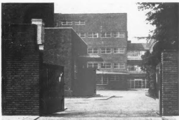
Above: one wing of the ward block; one of the entrances.
