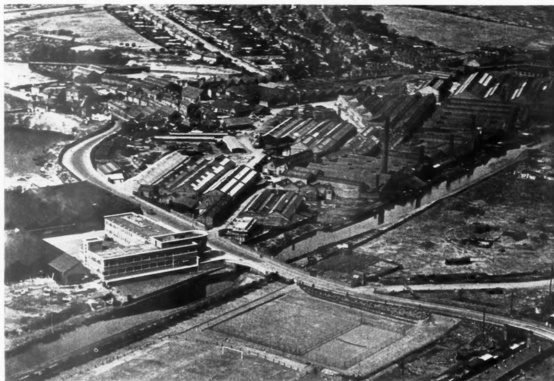
An industrial area near Birmingham, showing a steel tube factory and its new administrative offices on the left.
