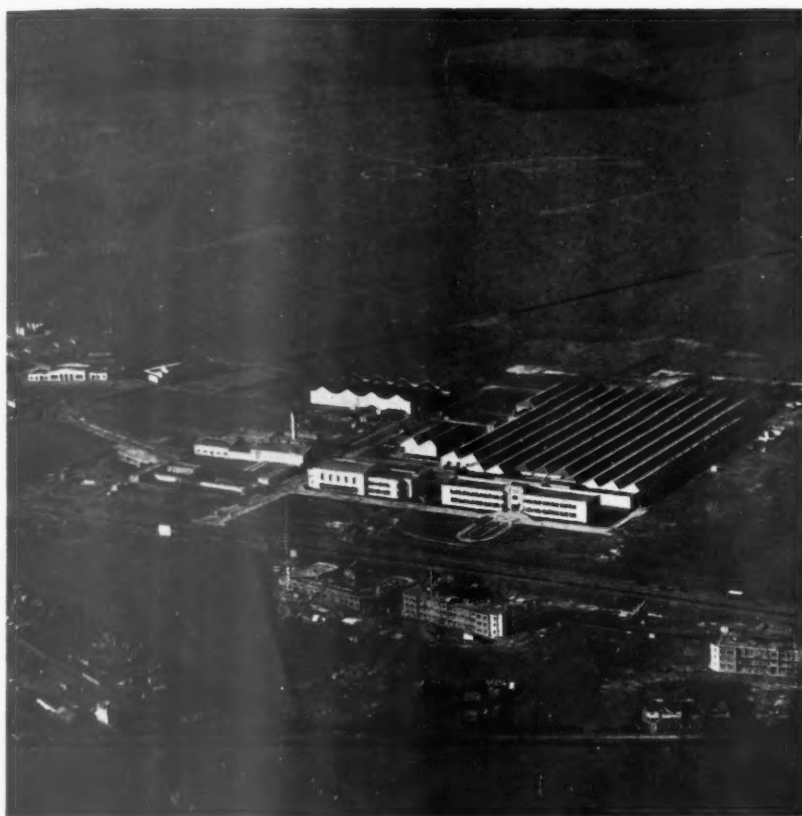
Factory building near the Barnet by-pass.
