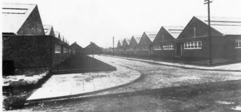
One of the blocks of sectional or unit factories at Welwyn. As a factory expands it can take over additional units and the standardized form brings economy in building costs. This type of unit is being used on new estates, and has great architectural, as well as commercial, possibilities.
