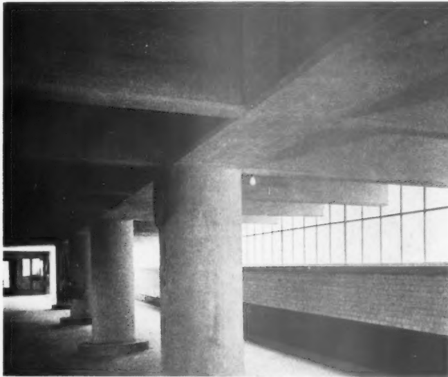
Axonometric, looking up, and photograph of reinforced concrete beam construction at the rear wall on an upper floor
