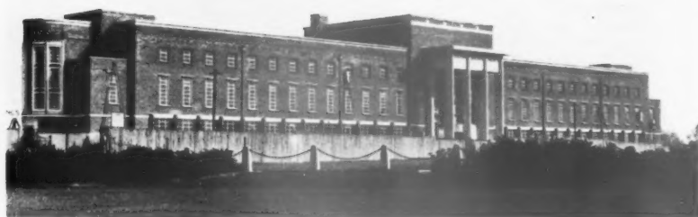
A progress photograph of Dagenham Municipal Buildings. Architect, E. Berry Webber.
