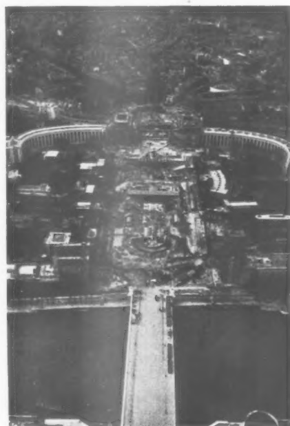
A progress photograph of the Paris Exhibition as seen from the Eiffel Tower.
