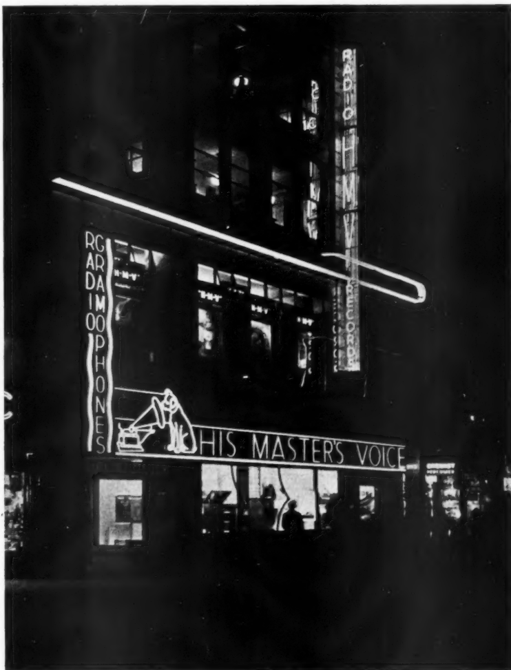
H.M.V. Gramophone Shop, Oxford Street. By Joseph Emberton. An example where neon lighting is a fundamental part of the design and not merely applied as an afterthought.
