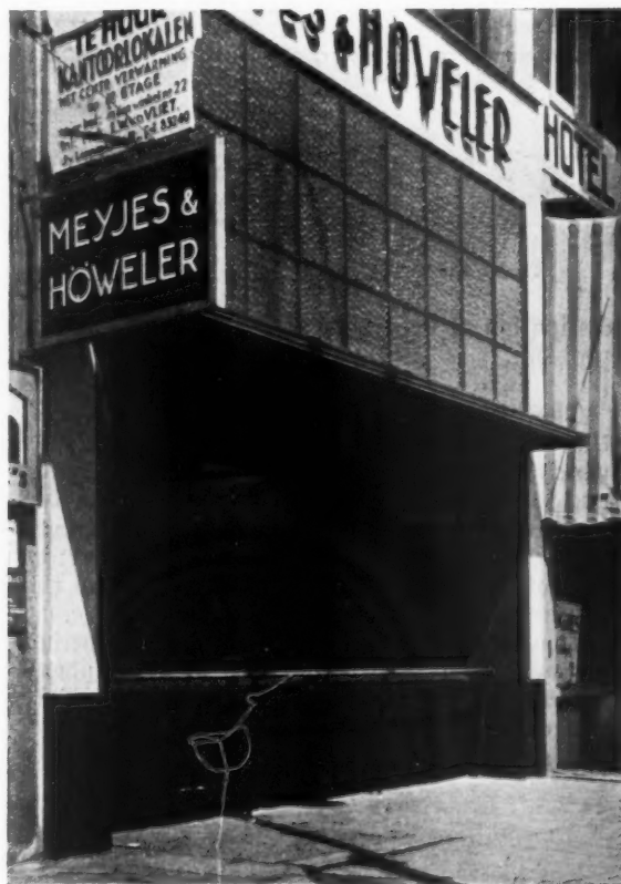
Above, a dress shop in Berlin, designed by O. R. Salvisberg; an example of first-floor windows used for display. Right, a cycle accessories shop in Amsterdam with a grey granite plinth, R.C. hood with granite aggregate bush-hammered finish, bronze guard-rail and supports and end walls of painted stucco.
