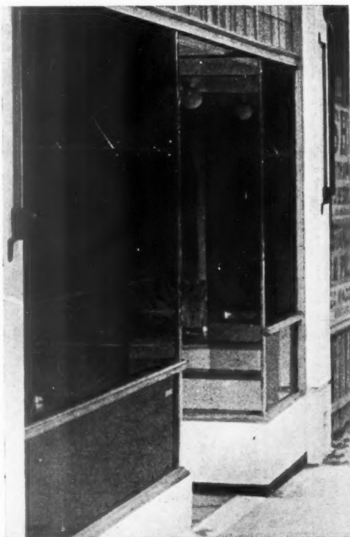
An example of the use of straight non-reflecting glazing combined with mirrors.
