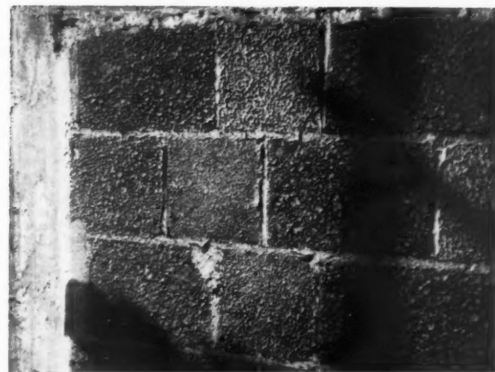
Above, the Fire Testing Station under construction, showing the reinforced concrete frame and the panel infilling of foamed slag blocks. On the right is a close-up of the blocks before rendering, showing the good key provided.
