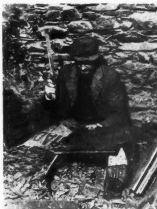
Above, shaping and dressing Westmorland slates with a straight-edge and hand knife. Left, drilling nail-holes; a modern development.
