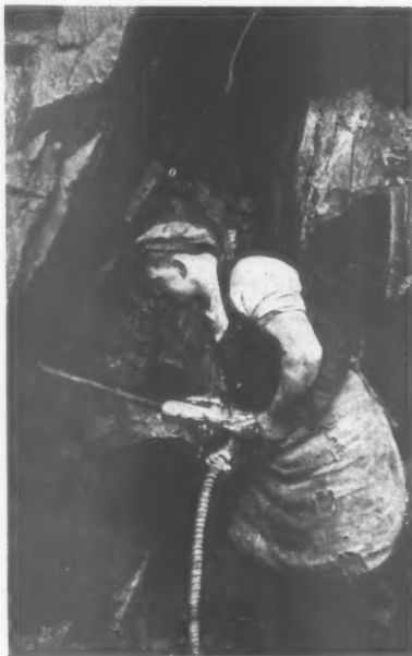
Drilling for a splitting charge in the Westmorland slate quarries.
