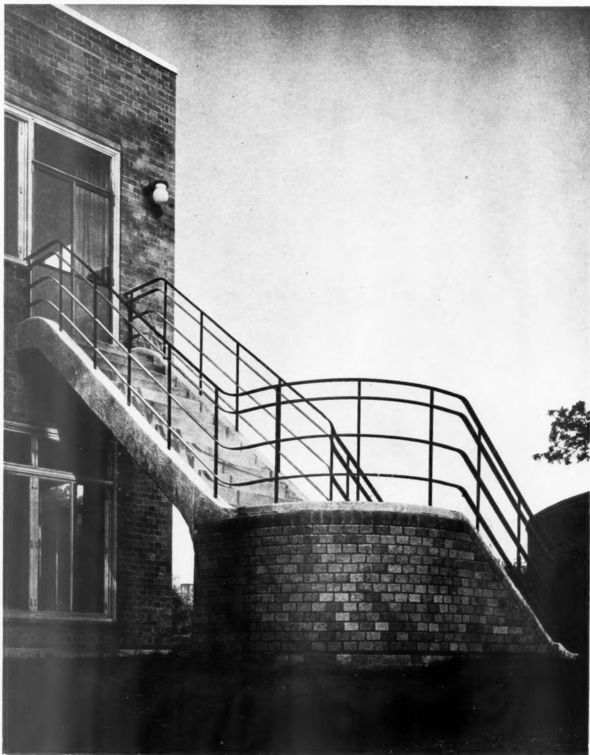
A brick and reinforced concrete escape stair with wrought iron balustrade. An axonometric and details are shown overleaf.
