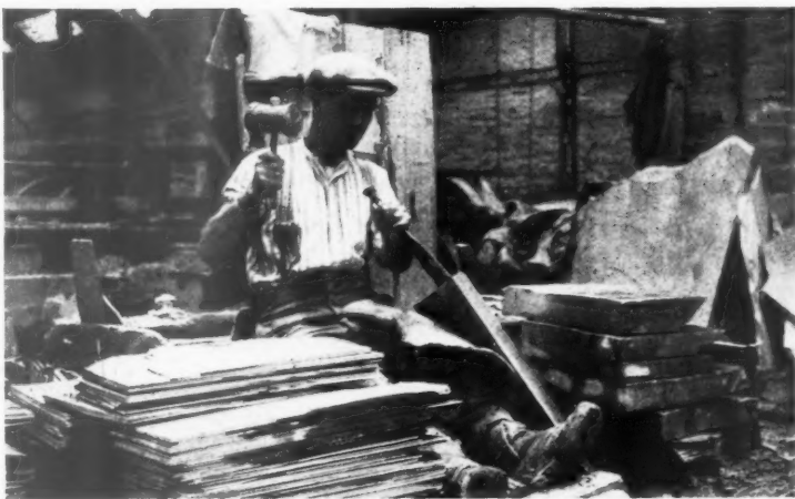
Splitting Delabole slates from the slabs.
