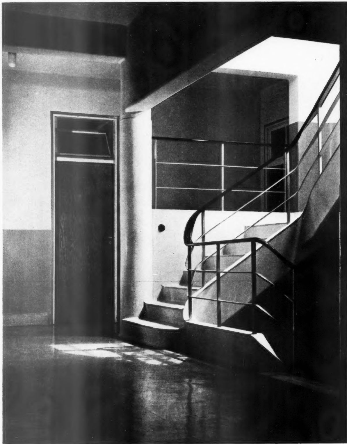
The staircase landing on the first floor. The walls and ceilings are executed in matt pale grey sirapite plaster and the dado is of oyster grey glossy enamel. The floor is covered with mottled green rubber and the staircase is of cream terrazzo. The wrought-iron railing, horizontal and raking bars are pale green and the vertical bars are blue-green. The door shown gives access to the nurses' station.
