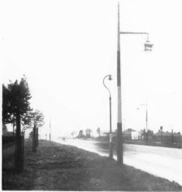
Adastra poles erected by the Rowley Regis Gas Company on the main Wolverhampton road. (See note below.)
