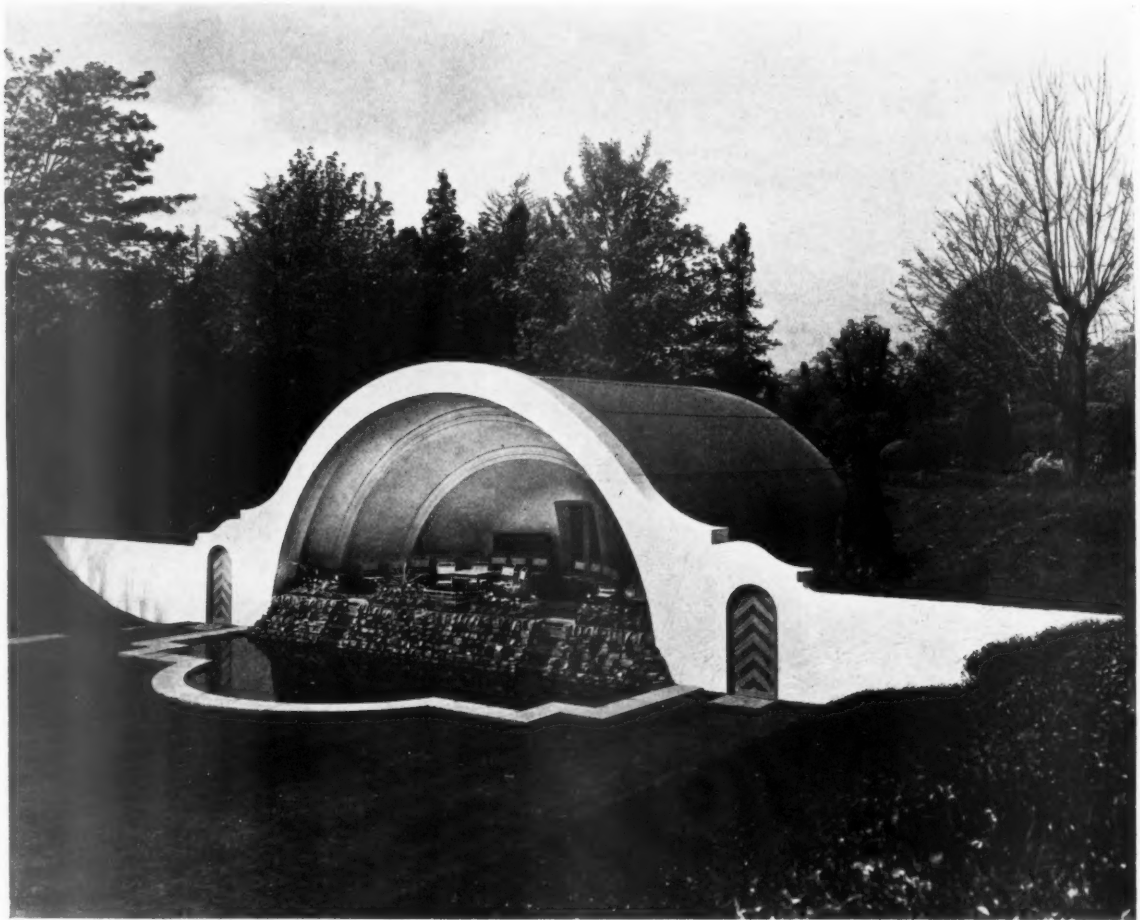
The bandstand illustrated above is covered with corrugated asbestos cement sheets. Inside, the stage lining is of asbestos cement with special asbestos troughs to carry strip lighting. Details of the design and construction appear overleaf.
