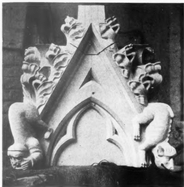
A piece of carving recently completed for one of the new pinnacles shortly to be placed in position on York Minster.
