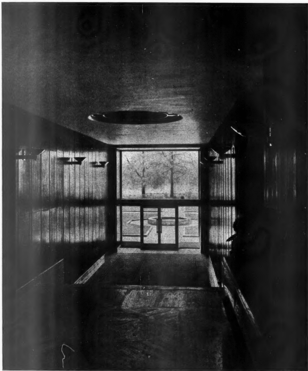
The light fitting shown in the drawings overleaf is an effective decorative feature in the entrance hall illustrated above. During the daytime light is admitted through glass bricks in the floor over, and at night it is lit indirectly by two lamps reflecting up on to the under-surface of the glass bricks. The bracket lamps seen on the walls provide the light necessary for ordinary purposes, the central light being mainly decorative. The fitting is carried out in obscured glass and wood finished with cellulosed aluminium paint.
