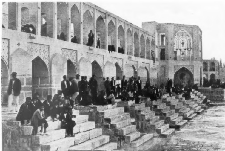
From the Exhibition of Photographs of Persian Architecture now being held at the R.I.B.A.: The Pulkhajoo Bridge, Isfahan.
