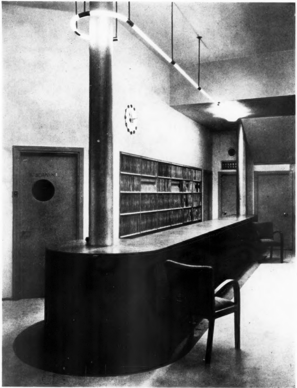
The counter illustrated above is designed for the sale of gramophone records, and the whole of the lower half is devoted to storage space. The counter is faced with walnut veneered plywood, and has a cork top. An axonometric and details are shown overleaf.
