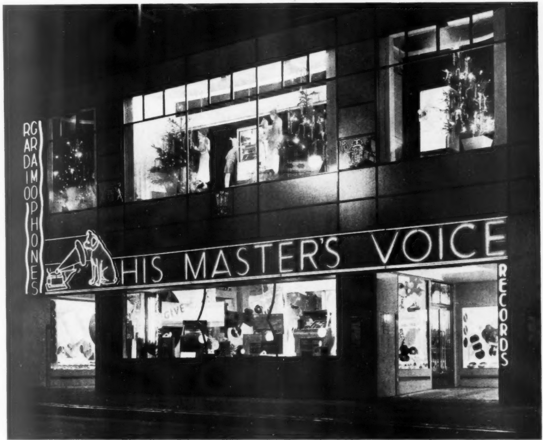
The shop illustrated above is designed for the display of gramophones and radio sets, and is provided with the now common non-reflecting glazing. The building is faced, up to second-floor level, with rough cast glass backed by building board. An axonometric and details are shown overleaf.
