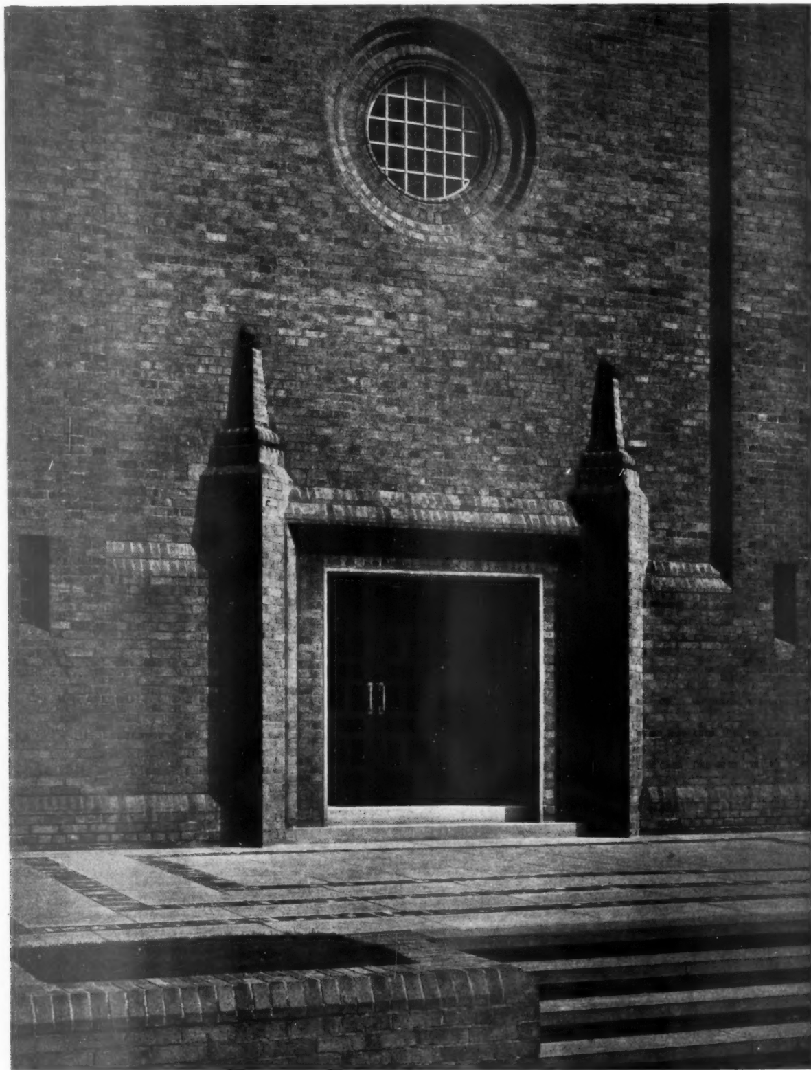
A detail of the west entrance and terrace, in warm yellow bricks and Ancaster stone.
