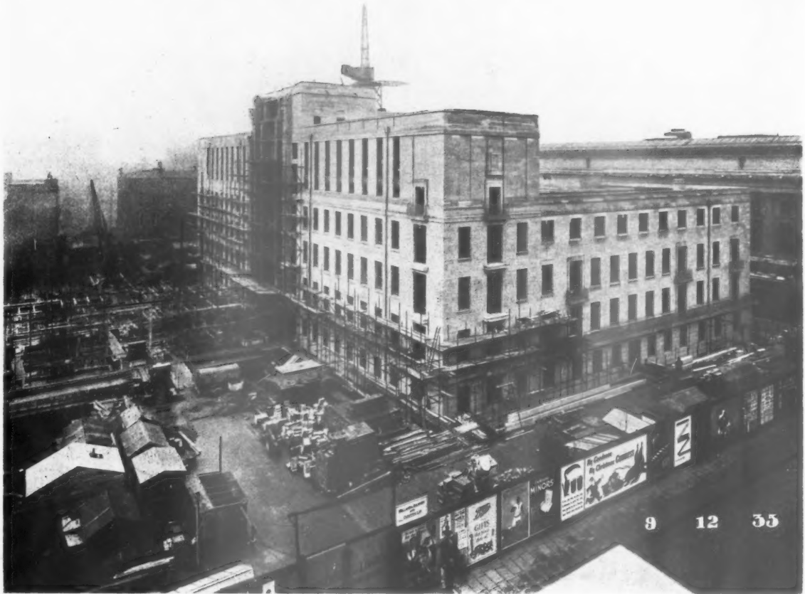
The building as it was a month ago. The steelwork for the main tower is up to first floor level, and the main lift hall is still open where it will ultimately connect with the tower. To the right is the north front of the British Museum.
