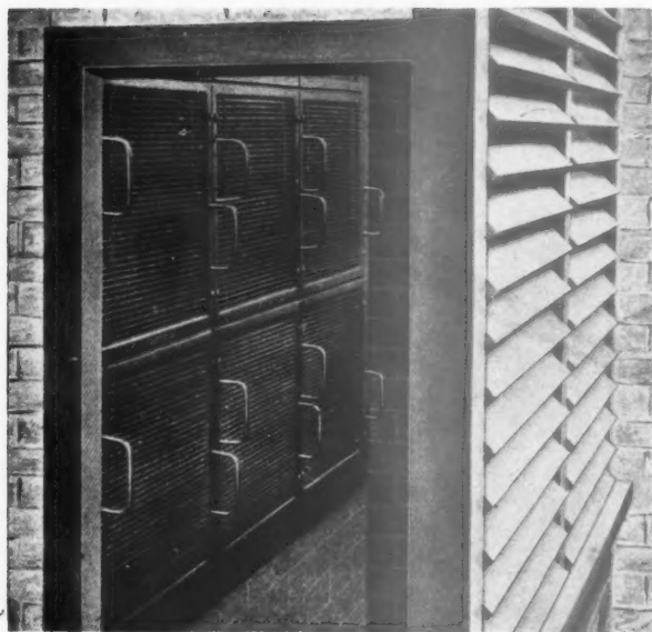
Figure 256. Typical oil-coated sectional air-filter.
