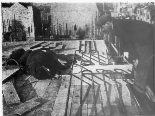
PROGRESS PHOTOGRAPHS. —Left, welding the heating coils, prior to their being cased solid in the floor slab concrete. Right, wiring the reinforcement on one lift of the wall-slabbing. On the left of the photograph is a window opening.
