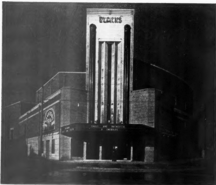
Walls of reconstructed stone and brick: black fluted flanking pilasters to central window, which is lined with stainless steel sheets, see detail drawing reproduced below. Blacks Regal Cinema, Newcastle-upon-Tyne. By Edwin M. Lawson.
