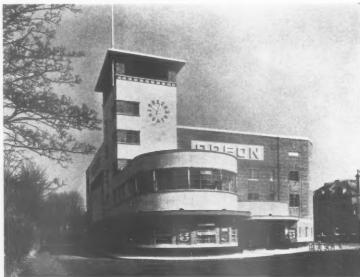
A combination of brick and terra-cotta, the last material being used as a decorative surface covering or veneer in tile-like form. Right, a detail of the central feature. Odeon, Worthing. By Whinney, Son and Austen Hall.
