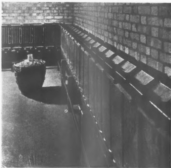
Storage batteries for the independent electric light supply. They are kept constantly charged by a rectifier, housed in a separate compartment. Their purpose is to provide an independent electric light supply in case of a breakdown in the main supply.
