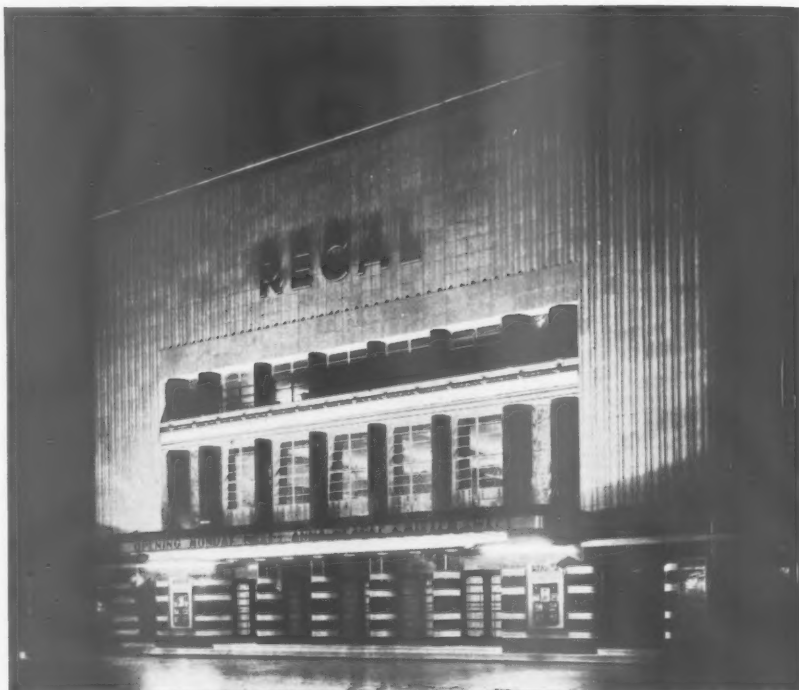
Reconstructed stone, with a granite finish; relieved by black faience columns to windows. Regal, Wimbledon. By Robert Cromie.
