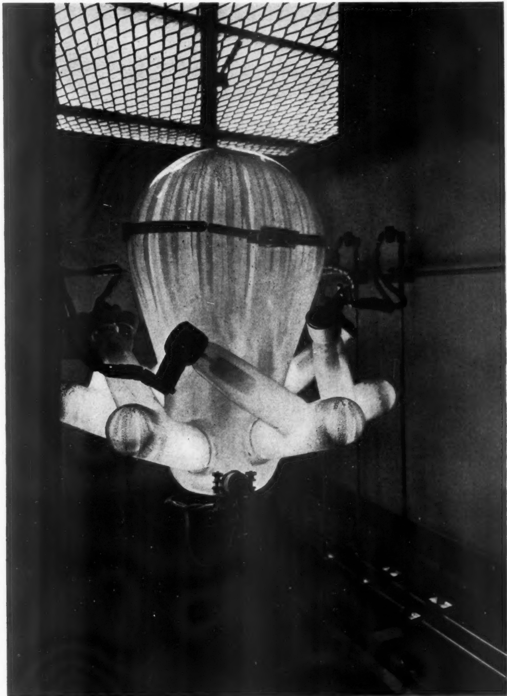
One of the two rectifiers. It charges the batteries used for the operation of the projecting machines and talkie apparatus; the other, the batteries for the independent electric light supply.
