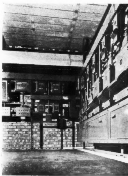
Part of the main switchboard in the large intake switch room.
