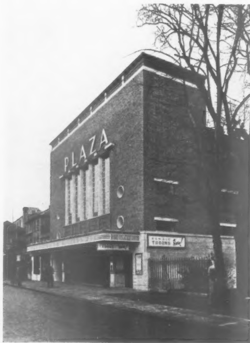
Two - inch multicoloured facing bricks with artificial Portland stone dressings. Plaza, Sutton. By Robert Cromie.
