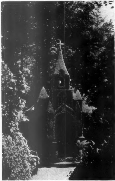
The Vauxbelets Chapel, Guernsey. This miniature chapel, built entirely by one man from material on the spot, is approximately 20 feet long and 15 feet high. It is a replica of the church at Lourdes. Pieces of broken china have been used for the "applied art" on the exterior.
