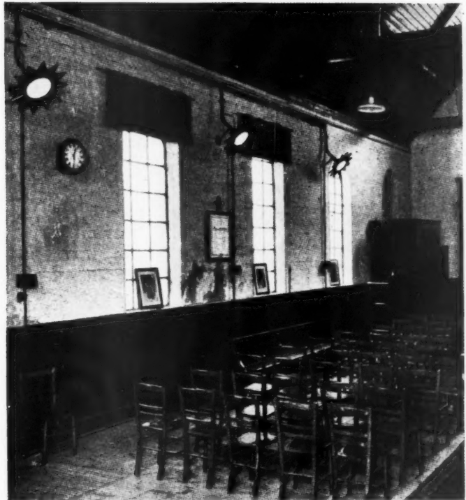
Figure 173. High temperature gas radiant heaters (Cox's).
