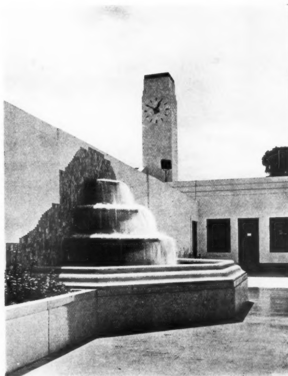
Cascade aerator used as a decorative feature in the end wall of a swimming pool. G. W. Smith, architect.
