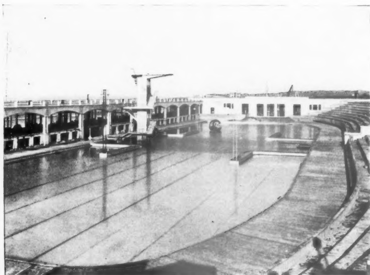
The Hastings pool, designed by S. Little. The surround is edged with non-slip carborundum tiles and is laid to a fall of 1 in 60 away from the bath.
