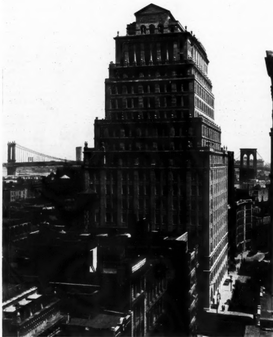
The Royal Building, New York. By Starrett and Van Vleck. A general view.
