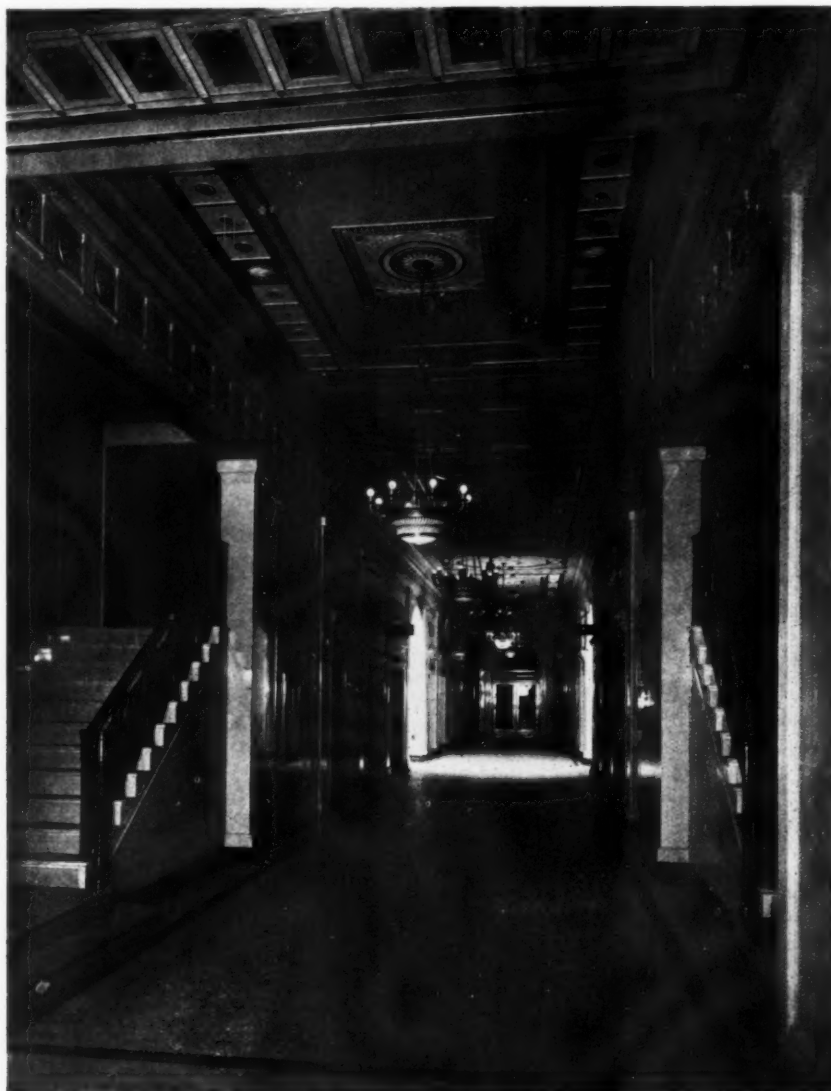
The Royal Building, New York. By Starrett and Van Vleck. The main floor, looking east.
