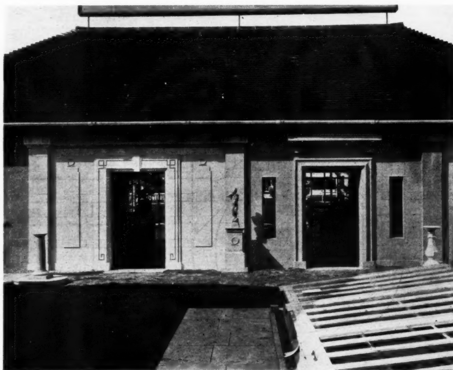
Part of the stand of Messrs. G. and T. Earl (1925), Ltd., and the Portland Cement Association, Ltd., at the Royal Agricultural Show, Nottingham.
