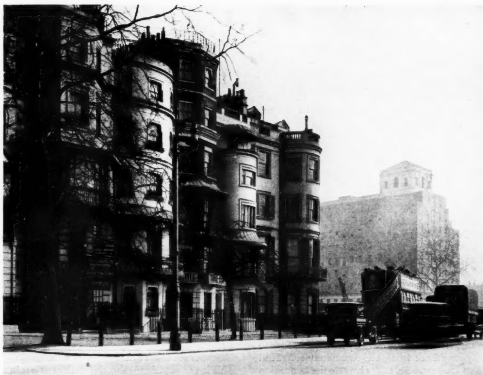
Park Lane, W. Above, a mansion rather on a scale with Belgravia than with Park Lane, and distinctly Italianate. Below, houses in Park Lane, showing Grosvenor House in the distance.
