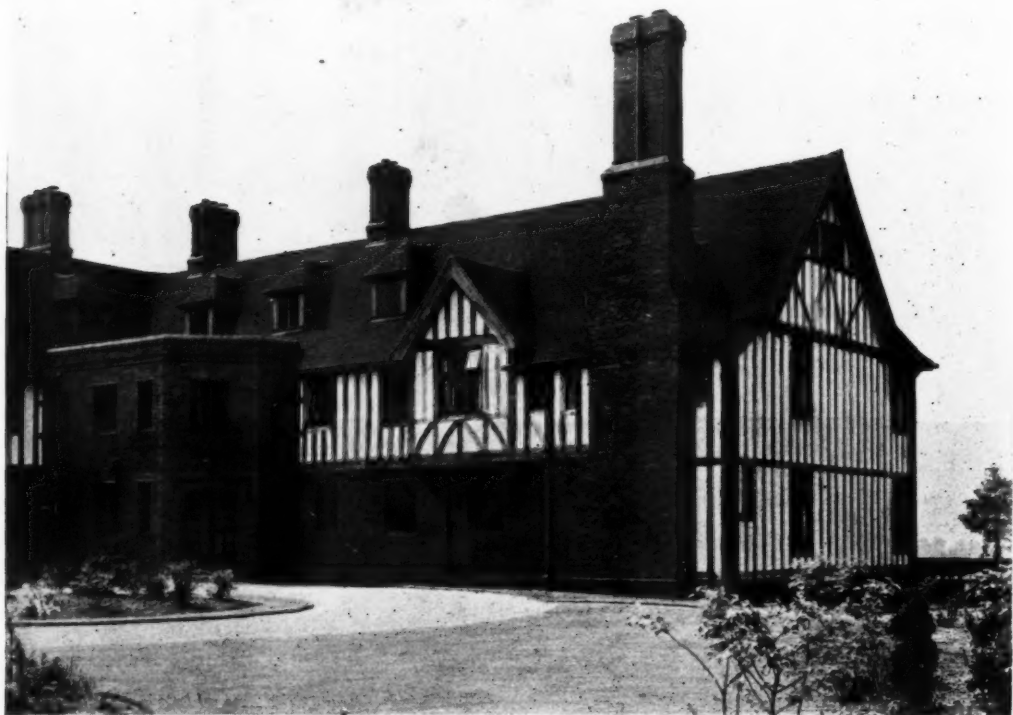
The Manor House, Stone, Worcestershire. By E. Stanley Hall. Above, the entrance front, from the drive. Below, the entrance and the north wing.
