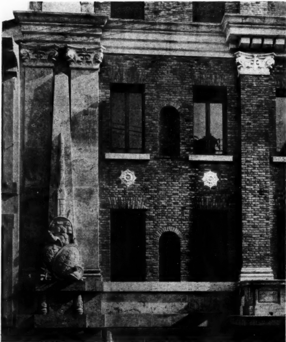
Fascist headquarters, Milan. By Colleoni. Detail of front elevation.
