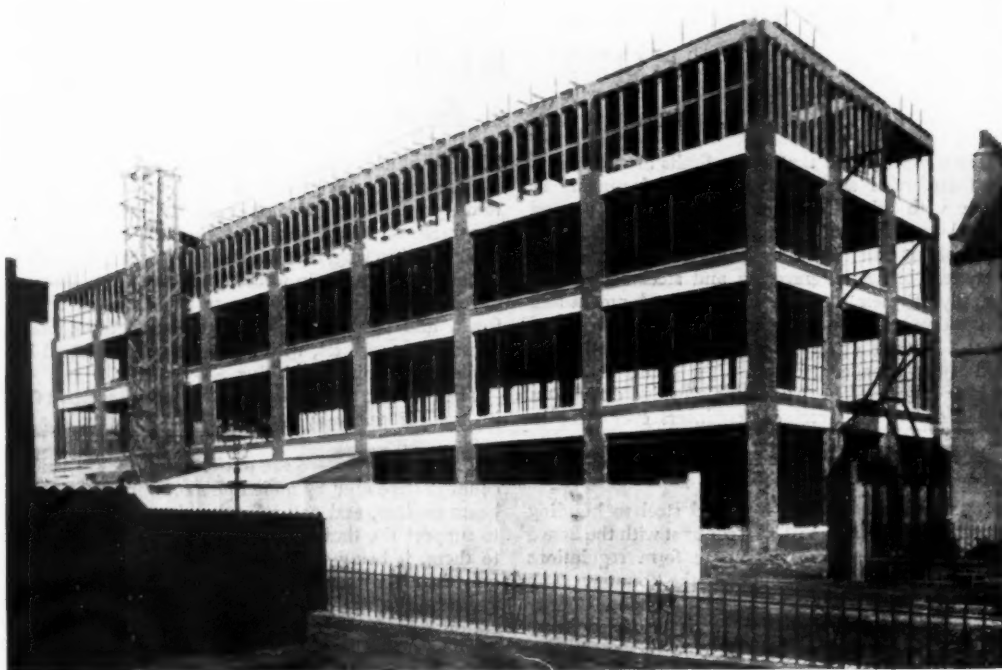
Figure two. A modern steel-framed factory building. [Compare the window area with that of figure one.]
