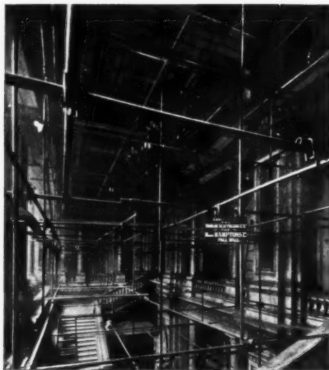
Scaffolding in the Foreign Office, London. By Scaffolding (Great Britain), Ltd.
