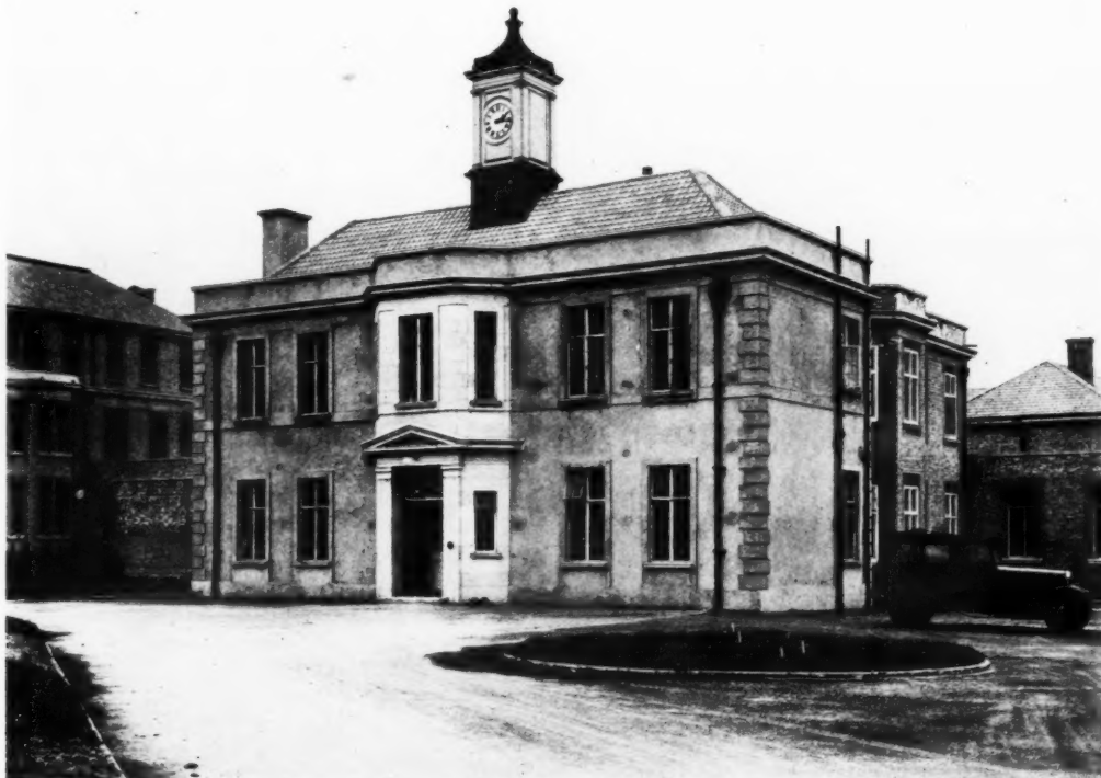
Redhill Hospital, Edgware. By Paine and Hobday. The administrative block.
