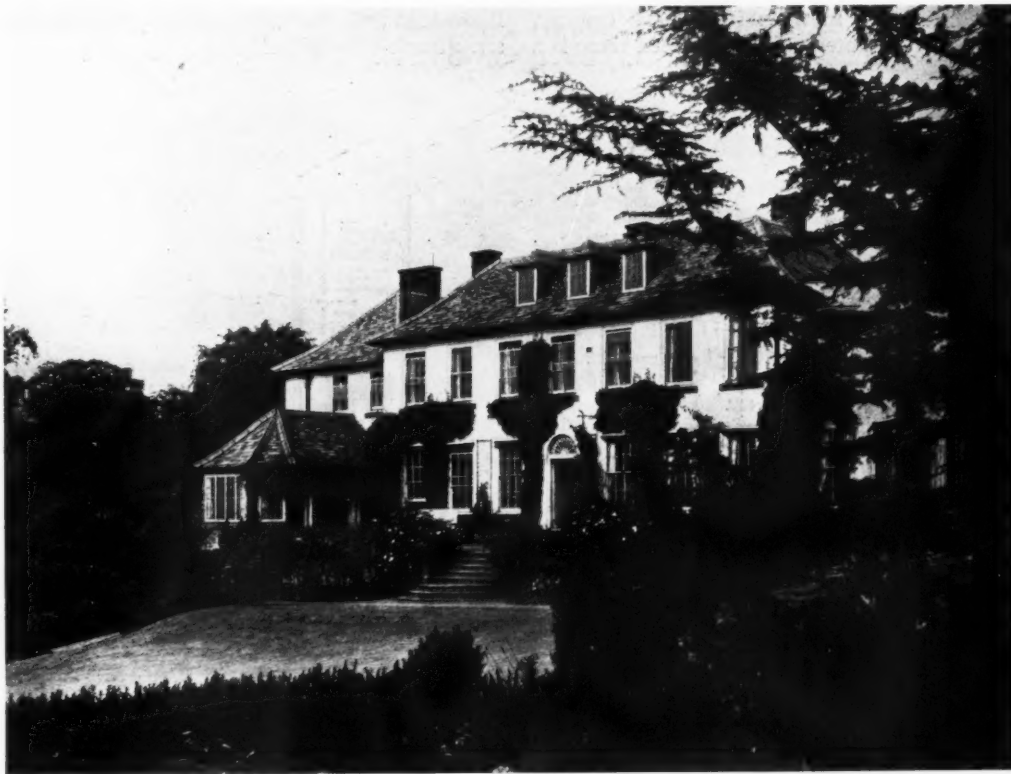
Stocktons, Alderley Edge, Cheshire. By Percy Scott Worthington. The garden side.
