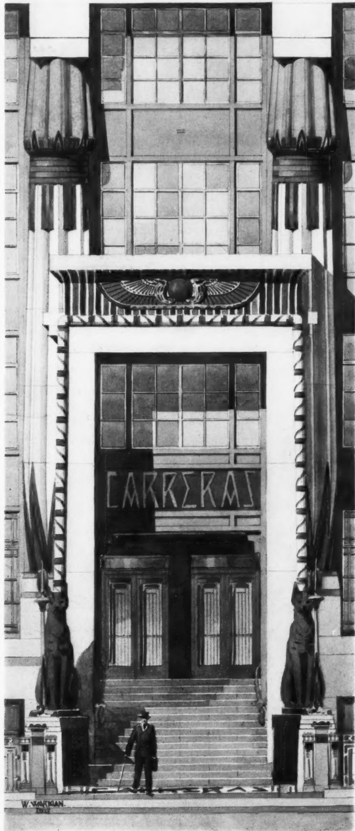
Detail of some of the "Atlas White" concrete in colour on the Carreras factory.
