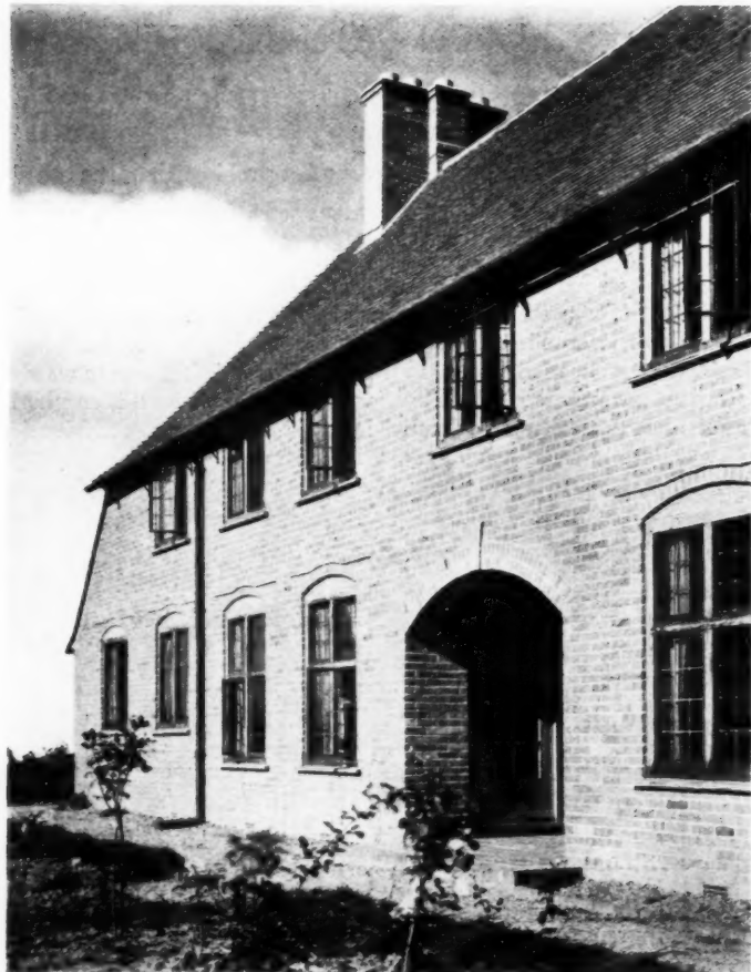
House at Chesham Bois. By Adams, Holden and Pearson. Two views of the garden side.
