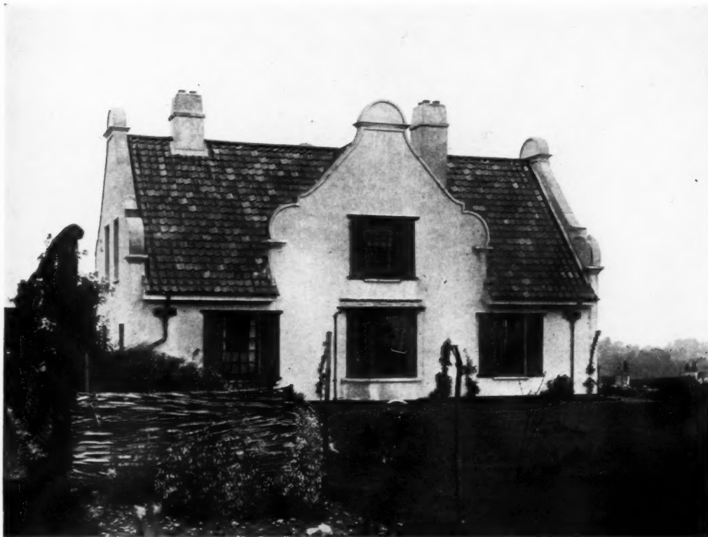
House at Budleigh Salterton, Devon. By Orphoot, Whiting and Bryce. Above, the south (garden) front
