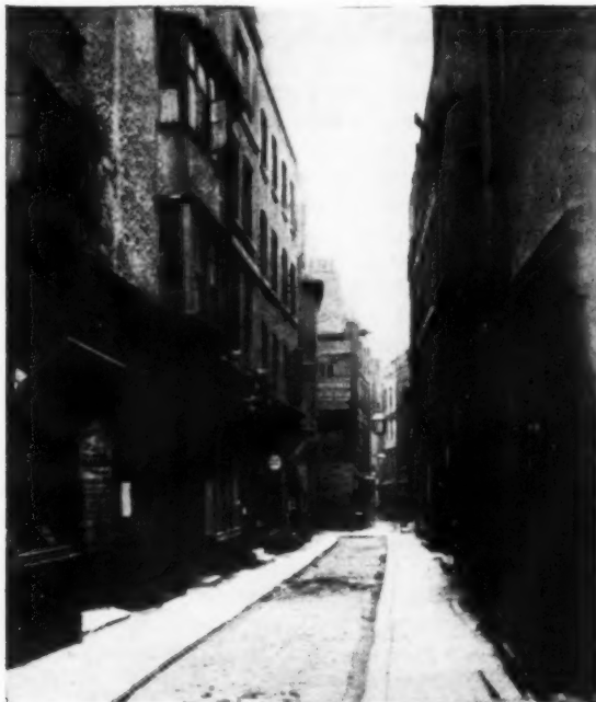
Bell Yard, Fleet Street.
