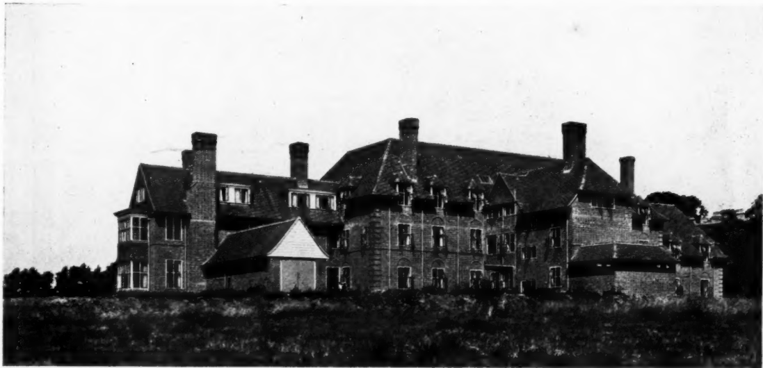
New buildings at Radley College, Berks. By H. I. Merriman and A. B. Knapp-Fisher. The house - masters' block.
