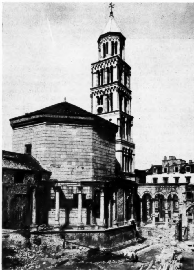
The cathedral and peristyle of Spljet. The columns and central dome form part of the Temple of Jupiter, afterwards the Imperial mausoleum. The columns are of various stones, many having been brought from Rome and Egypt. The tower was added last century, and, from the Roman point of view, is an anachronism. It is after the style of an old bell tower at Rab, and was put up by the English architect, Jackson.
