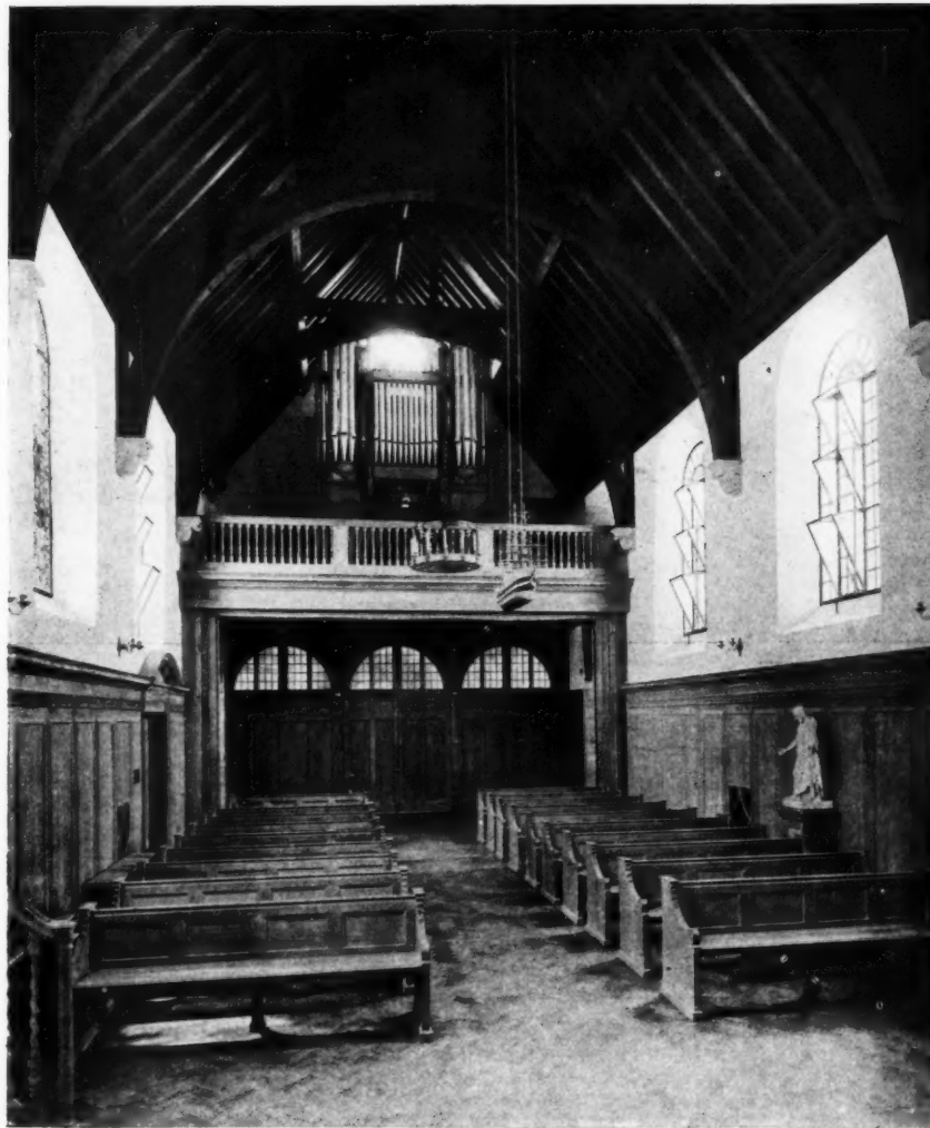
Norwegian Sailors' Institute and Church, Rotherhithe. By John L. Seaton Dahl. Above, the church, looking from the altar. Below, reading from left to right, ground-floor, basement, gallery, and first-floor plans.
