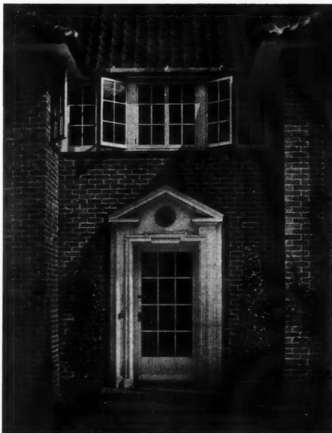
Quietways, Brasted Chart, Kent. By Oswald P. Milne. Above, a general view. Below, the entrance door.
