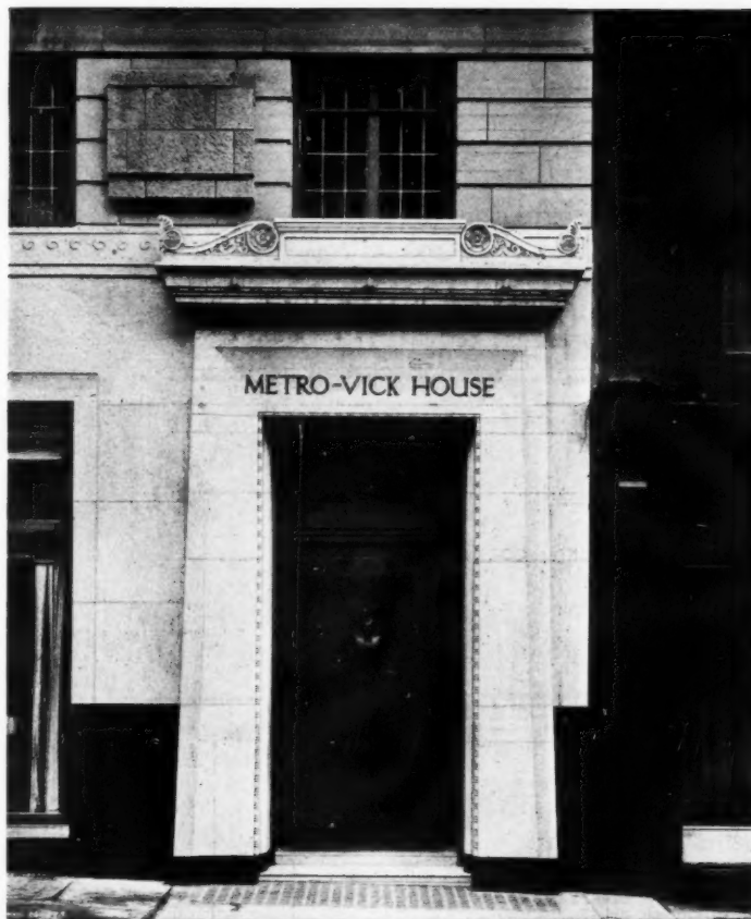
[A working detail of this entrance doorway appears on the following page]
