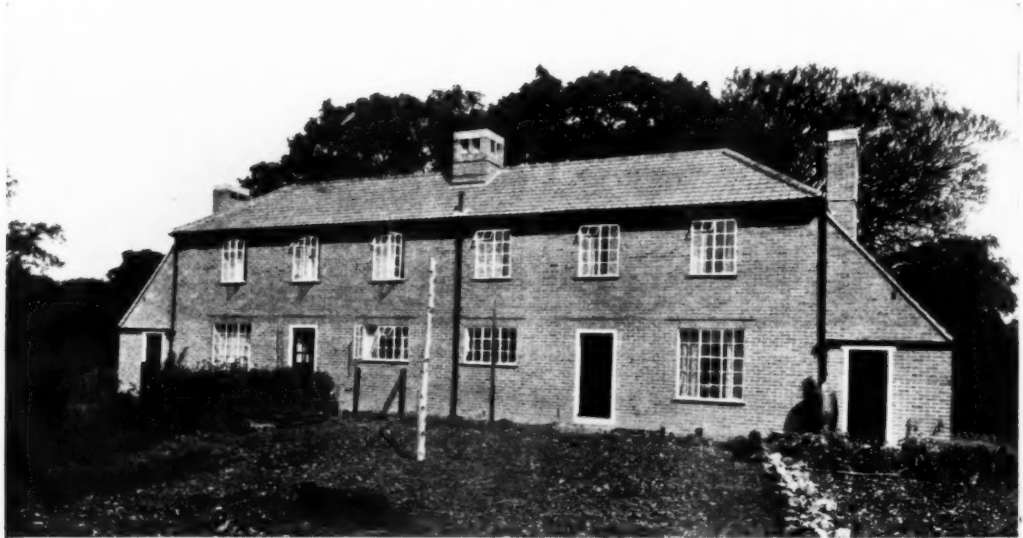
Above, house at Clevedon, Somerset. By C. F. W. Dening, and centre, left, the plan. Below, pair of cottages at Potten End, Hertfordshire. By W. B. Hopkins, and centre, right, the plan.
