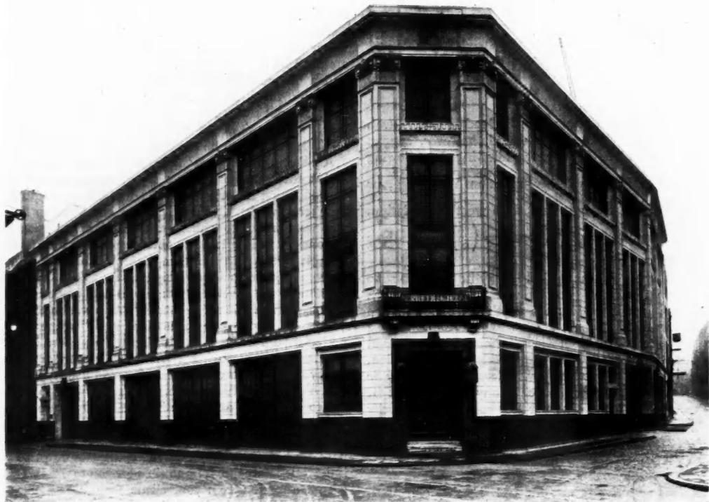
Northcliffe House, Tudor Street, London. By Ellis and Clarke. A general view.
