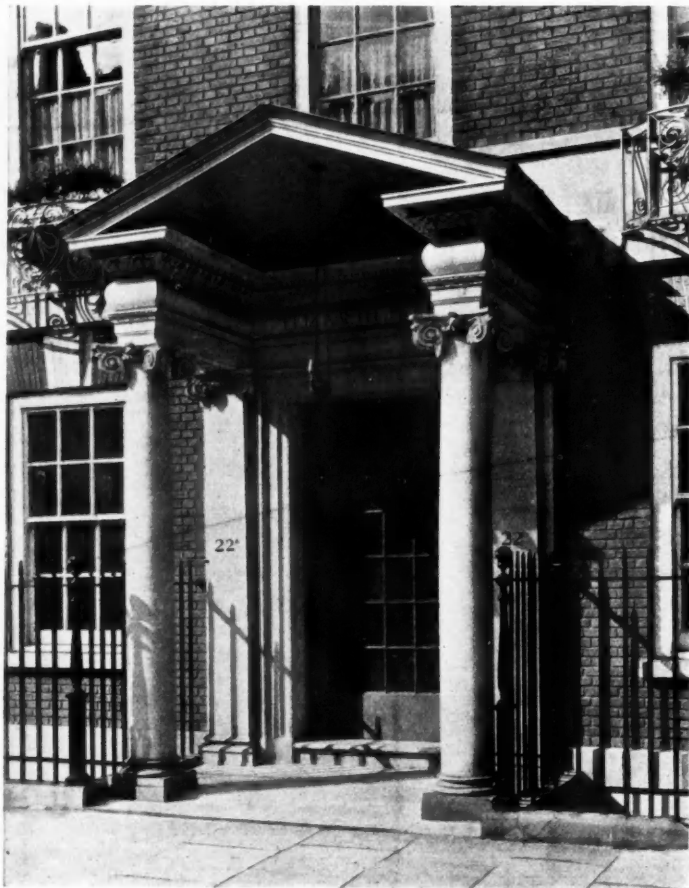
The Elizabeth Fulcher Nursing Home, Devonshire Street, London. By James J. S. Naylor. Above, a detail of the Devonshire Street front. Below, the main entrance.
