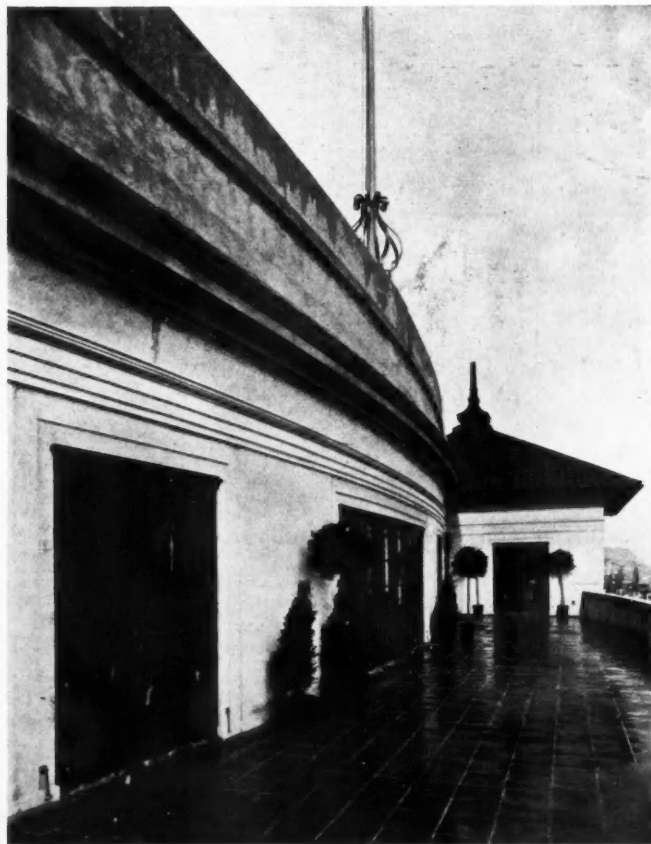
The White Rock Pavilion, Hastings. By Charles Cowles- Voysey and the late Hugh T. Morgan. Above, the tea- room on the ground floor. Below, the open promenade.
