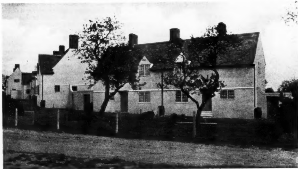
Cottages at Debden, Essex. By Kieffer and Fleming. [From Cottages: Their Planning, Design, and Materials.]
