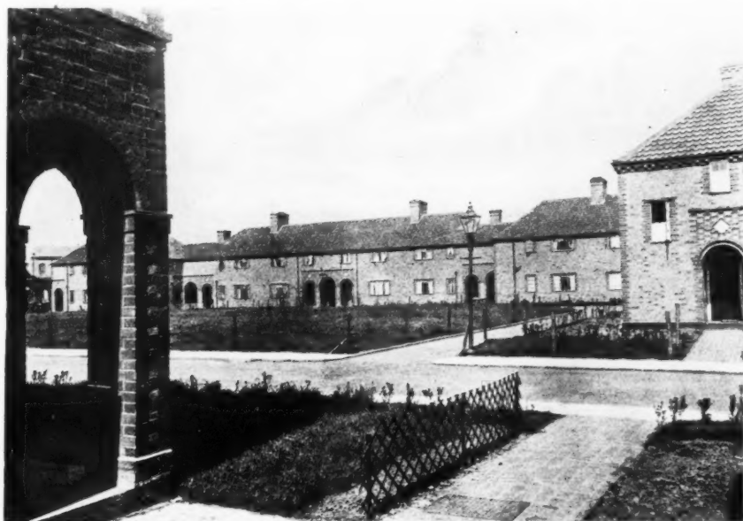
Square in Clematis Street, Hammersmith. By Matthew J. Dawson. [From Cottages: Their Planning, Design, and Materials. ]
