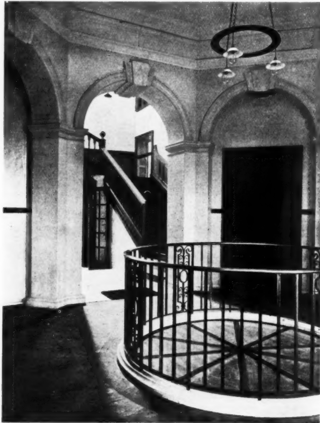
Oxford School of Pathology. By Edward Warren. Octagonal centre hall, looking south into main entrance hall, with circular floorlight in centre.
