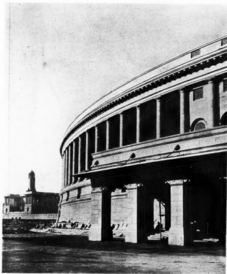
The new capital at Delhi. The legislative chamber. By Sir Herbert Baker. Above, part of encircling colonnade and porch. Below, a detail of the porch, with the secretariat building in the distance.
