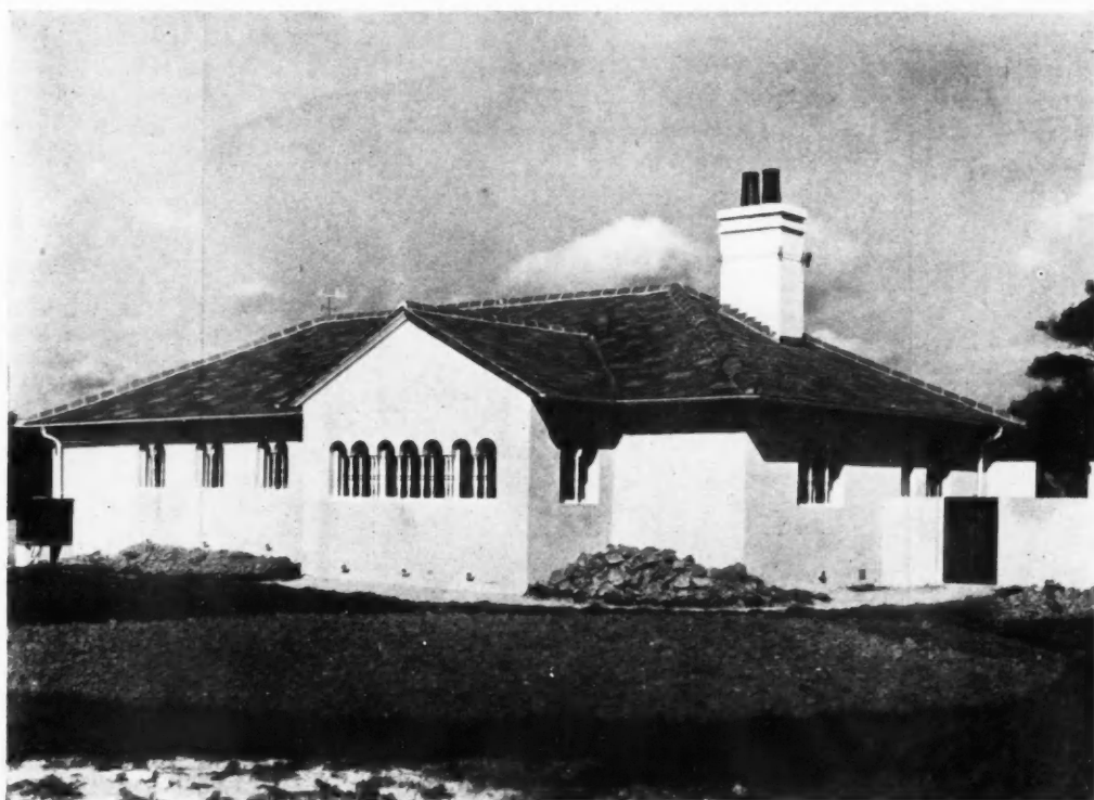
Ockdens, Birdham, Chichester. By John D. Clarke. Above, the south front. Below, another view of the same front.
