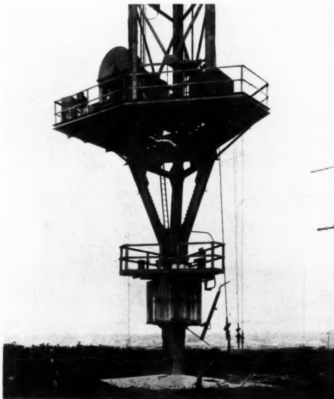
The Rugby Imperial Radio Station. By F. A. Llewellyn, O.B.E. Above, the entrance gates from Watling Street. Below, the base of one of the 820-ft. masts. Each mast has a lift inside its shaft to carry three men.
