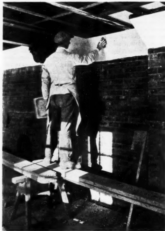
Left, figure four. Cutting out irregularities from the edge of the plastered surface where it adjoins brickwork purposely left to show in the interior. Right, figure five. Working up a texture on the lime putty finishing coat with the "wooden float." The edges are trimmed and the smudges cleaned off as separate operations.
