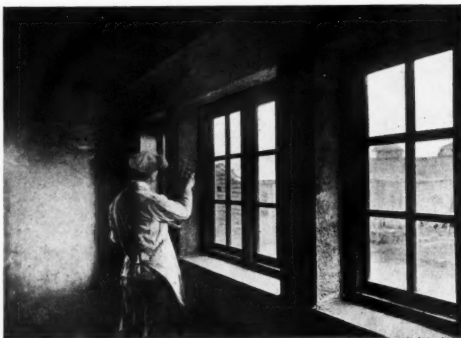
Figure three. Using the steel "laying trowel" to form the Portland cement rendering coat on the window reveals. By using this trowel a reasonably straight angle is obtainable.
