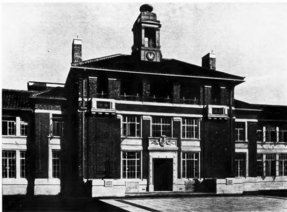
King George V Secondary School for Boys, Southport. By W. F. Granger and J. R. Leathart. Above, the south front from Scarisbrick New Road. Below, a detail of the central administrative portion of the south front.
