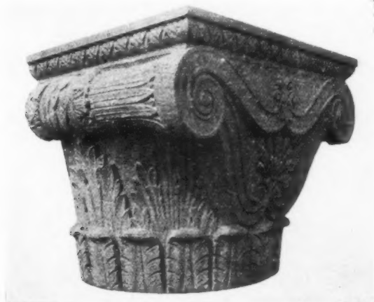
Worthing pier pavilion. Detail of caps to exterior columns round entrance hall.
