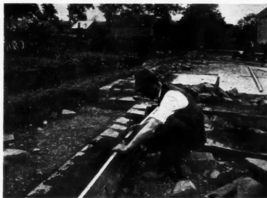
Figure four. The level of the newly-bedded stone is tested with a straight-edge and a spirit-level. Another spirit-level is seen on the ground to the right and a piece of curved walling in the background.
