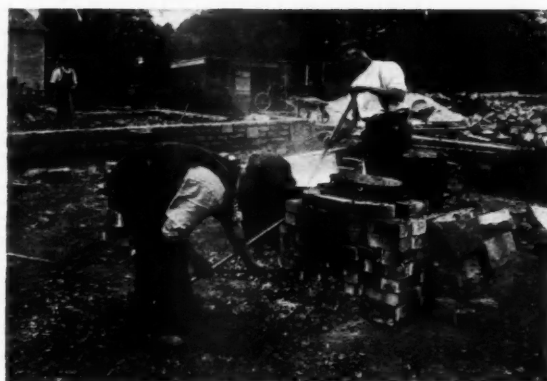
Figure six. Heating and mixing the materials for the damp-proof course, asphalt and gravel, in iron cauldrons over an improvised furnace which also heats the asphalted iron bars. A view of the stone facings appears in the background.
