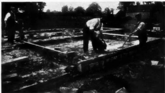
Figure five. The asphalt damp-proof course in process of application. The edge of the portion already laid has been splay rebated to avoid a straight vertical joint between two layings of asphalt. Masons are at work on the brick partitions and fireplaces.
