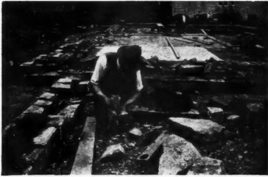
Left, figure two. Hammer dressing a backing stone. The stone is reduced to its dimensions by removal of successive flakes with the edge of the cutting hammer. The mason's line is supported in position by winding it round a brick placed at the correct level. Right, figure three. Packing small pieces of stone into a bed of mortar between the facing and backing stones of the wall. A bed of mortar is afterwards spread over the top of these spalls and across the tail ends of the larger stones.
