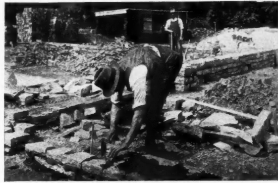
Left, figure two. Hammer dressing a backing stone. The stone is reduced to its dimensions by removal of successive flakes with the edge of the cutting hammer. The mason's line is supported in position by winding it round a brick placed at the correct level. Right, figure three. Packing small pieces of stone into a bed of mortar between the facing and backing stones of the wall. A bed of mortar is afterwards spread over the top of these spalls and across the tail ends of the larger stones.
