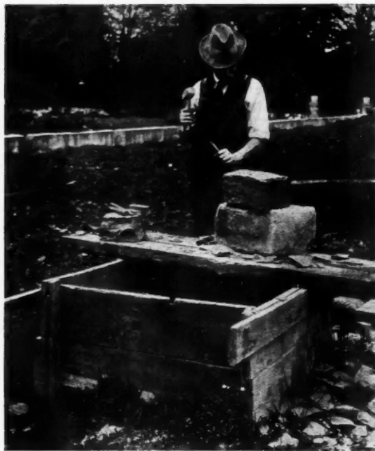
Figure one. Using the "point" to remove roughnesses from the upper bed of a facing stone. A "banker" has been improvised with a block of soft Bath stone and a pair of planks.
