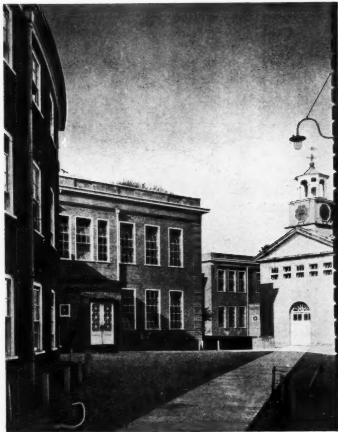
The new buildings at Stowe. By Clough Williams - Ellis. Above, classroom blocks, numbers 2 and 3. Below, the new buildings within the East court — study block and classrooms.
