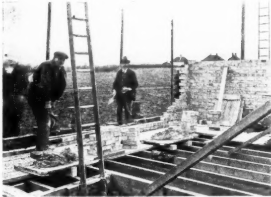
Left, figure two. The interval between the completion of the bricklayers' work on the ground floor and the commencement of operations on the first-floor walls has been reduced to a minimum by the use of lintols prepared for immediate insertion in the work at the proper height. Right, figure three. The built-up corners of the side walls are used as supports for the bricklayers' lines. Plentiful supplies of mortar of the right consistency, not too fluid, are necessary for speedy work.
