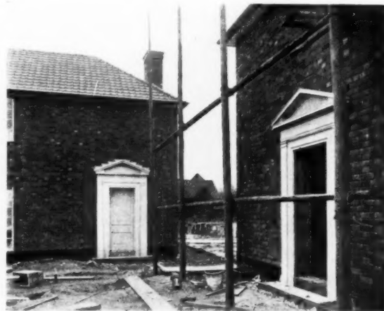
Figure one. Cottages at Welwyn Garden City. Economy has been considered in the plain, square plan and level eaves, which facilitate the bricklayers' work.
