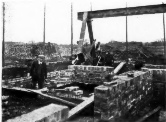
Left, figure four. The bricklayers have been stopped for the laying of a sound asphalt dampcourse, but in other respects straightforward working has been considered. The girder is temporarily supported on a wooden trestle in order that the steelworker need not return to fix a single connection. Right, figure five. The different colours of the Fletton bricks used in backings will be covered with plaster, but the question is raised whether a finer brick used inside and left exposed is not also a legitimate way of treating brick construction.
