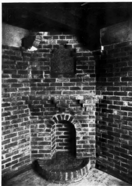
Figure six. Brickwork used in the interior of a dwelling-house. The fireplace will be darkened with smoke to carry the colour-note of the beams, and the panel above will be filled with antique tiles.
