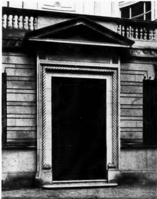
The main entrance. By Mewès and Davis.
