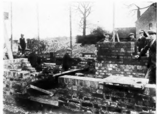
Left, figure four. The bricklayers have been stopped for the laying of a sound asphalt dampcourse, but in other respects straightforward working has been considered. The girder is temporarily supported on a wooden trestle in order that the steelworker need not return to fix a single connection. Right, figure five. The different colours of the Fletton bricks used in backings will be covered with plaster, but the question is raised whether a finer brick used inside and left exposed is not also a legitimate way of treating brick construction.
