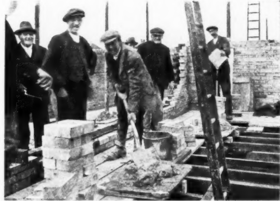
Left, figure two. The interval between the completion of the bricklayers' work on the ground floor and the commencement of operations on the first-floor walls has been reduced to a minimum by the use of lintols prepared for immediate insertion in the work at the proper height. Right, figure three. The built-up corners of the side walls are used as supports for the bricklayers' lines. Plentiful supplies of mortar of the right consistency, not too fluid, are necessary for speedy work.
