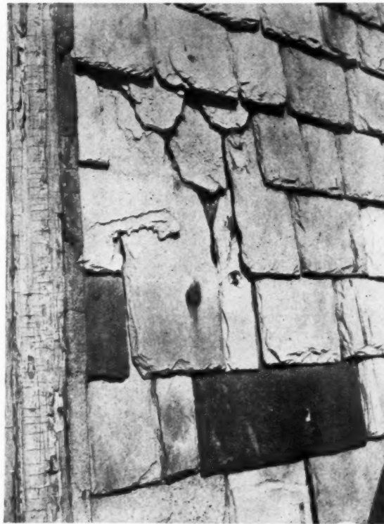
Green Westmorland slates on dormer cheek at Chelsea Hospital.
