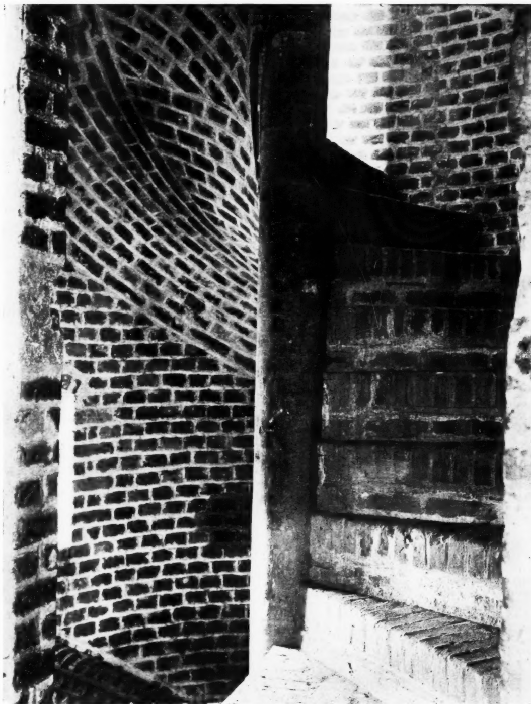
Brick newel stair with moulded brick handrail, in Essex Faulkbourne Hall (before 1494). (From A History of English Brickwork.)
